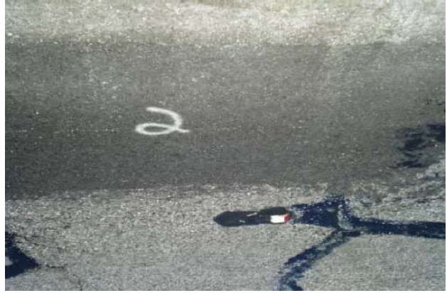
Figure 45. Patch 2 on Site IH410-1.
