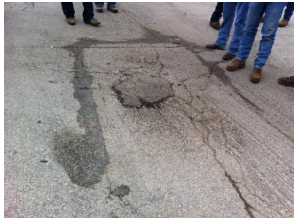
Figure 8. Water after Unit Removal.
