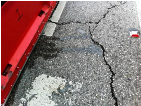
Figure 7. Condensed Water along Unit.
