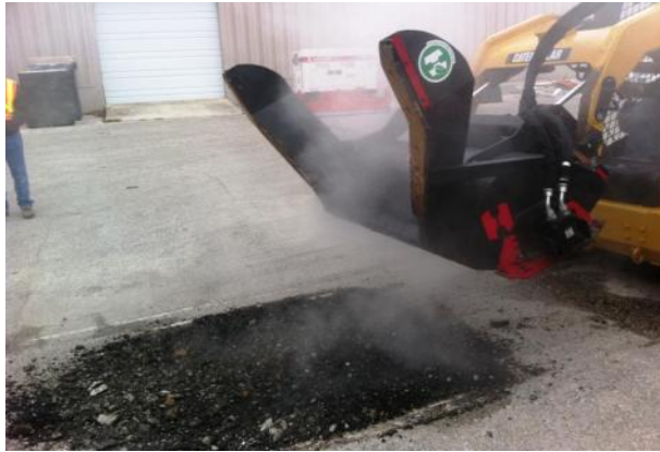
Figure 16. Preparing to Mill and Scarify.
