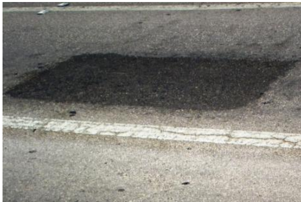
Figure 48. Patch 5 on Site IH410-2.
