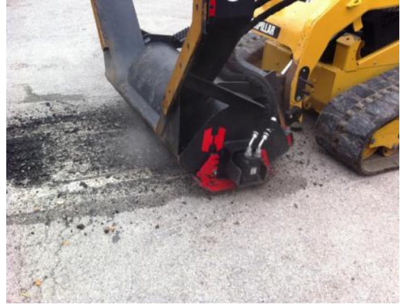
Figure 14. Milling and Scarifying.
