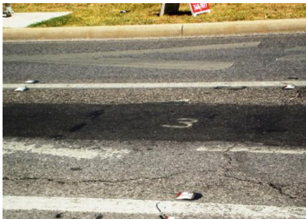
Figure 46. Patch 3 on Site IH410-2.
