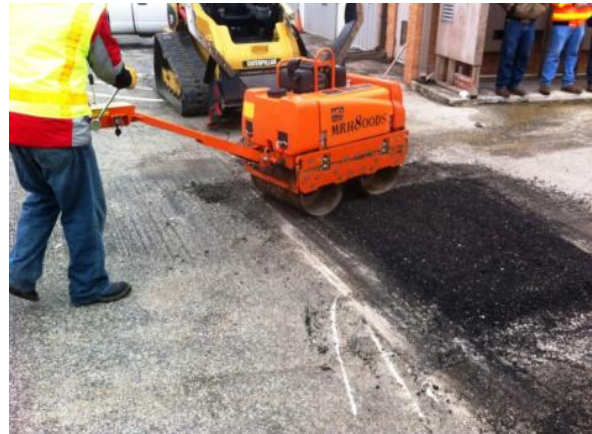
Figure 21. Rolling Finished Patch.
