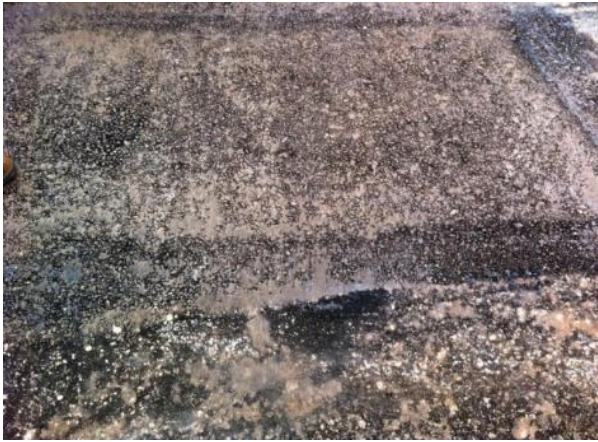
Figure 22. Completed Patch
