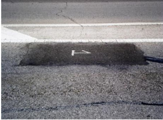
Figure 44. Patch 1 on Site IH410-1.
