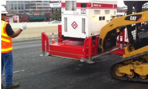
Figure 3. Unloading Generator and Heater.
