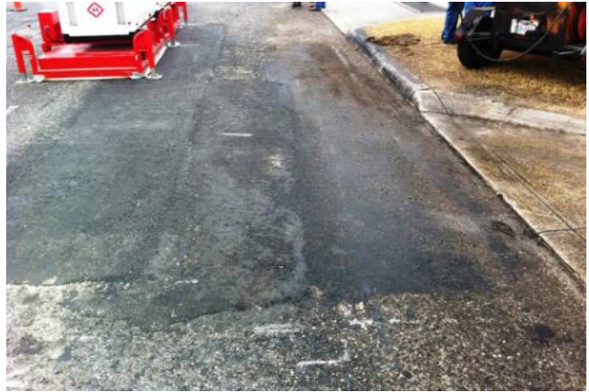
Figure 23. Multiple Patches and Overlap.
