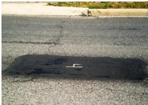
Figure 47. Patch 4 on Site IH410-2.
