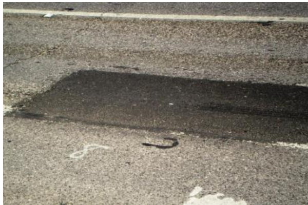
Figure 49. Patch 8 on Site IH410-2.
