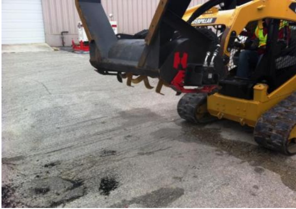
Figure 13. Preparing to Mill and Scarify.
