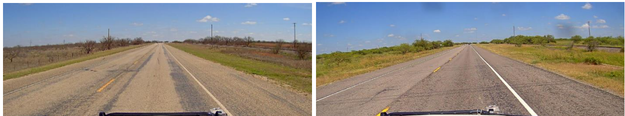
Figure 5. US 67 EB Surface Conditions: Before (Left) and After (Right) Seal Coat.
