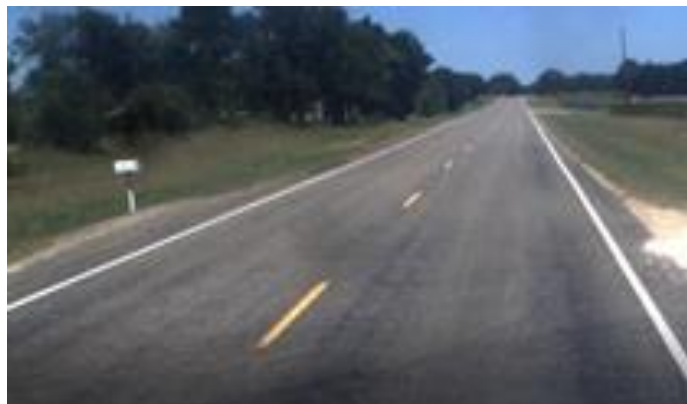
Figure 11. FM 1915 NB Surface Conditions: After Seal Coat.
