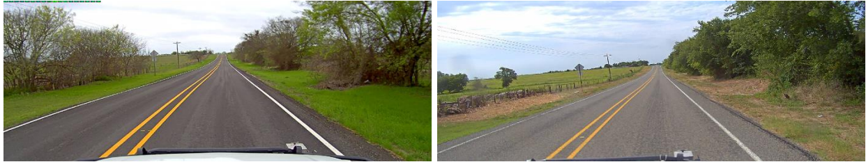
Figure 7. FM 339 SB Surface Conditions: Before (Left) and After (Right) Seal Coat.
