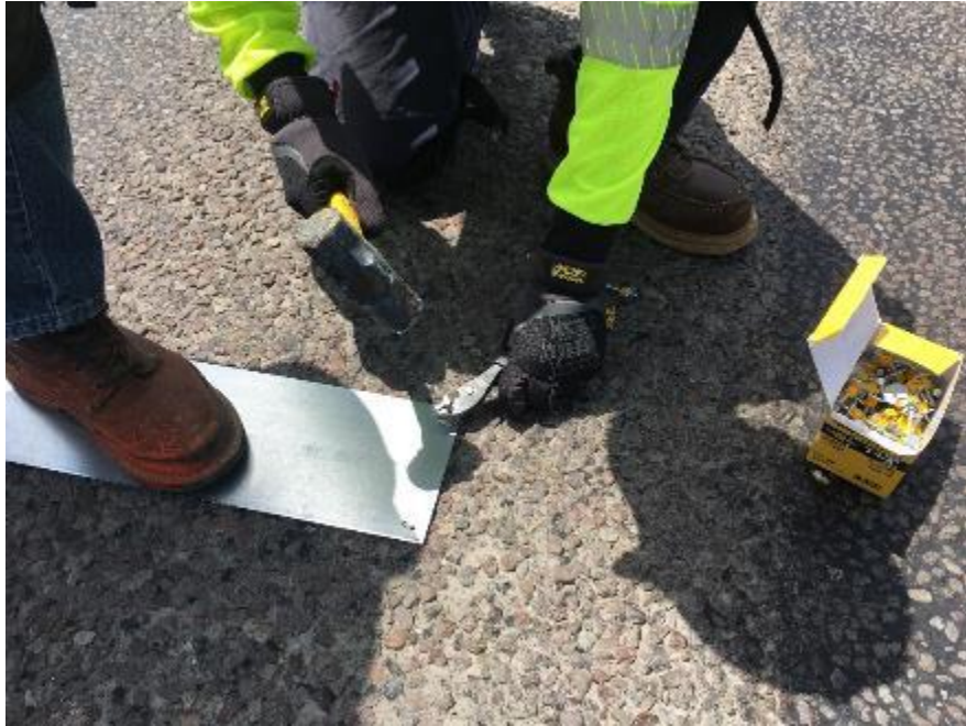
Figure 36. Nailing the Metal Plates.
