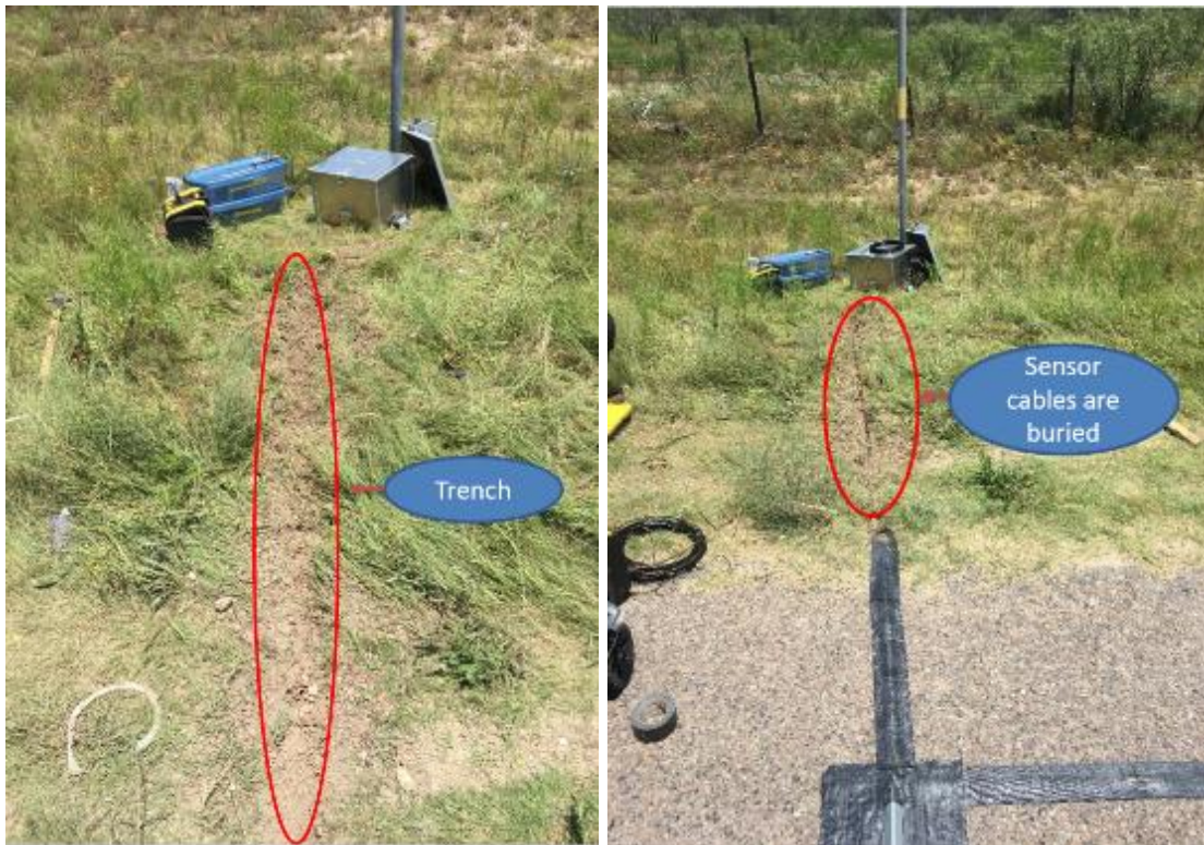
Figure 45. Sensor Cables Are Buried in Trench.
