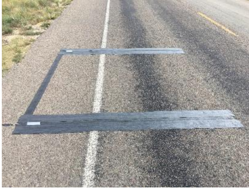
Figure 42. 6-Inch Road Tape Applied on the Pavement.
