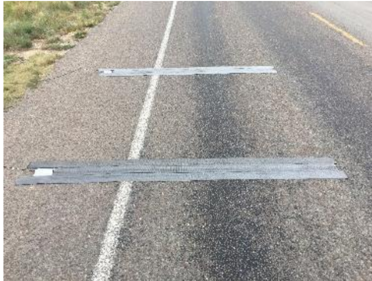
Figure 40. 4-Inch Road Tape Applied on the Pavement.
