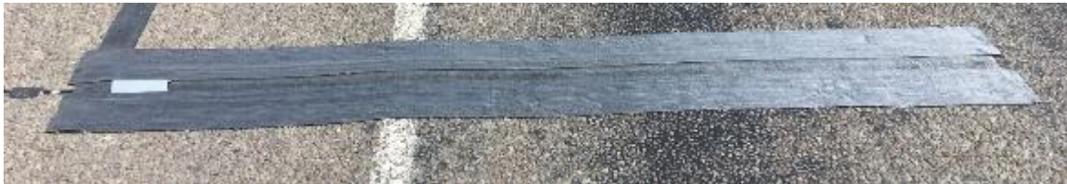
Figure 15. 6-Inch Road Tape Installed on the Road.
