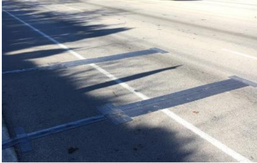
Figure 24. Portable WIM Installation on US 290 in Travis County.
