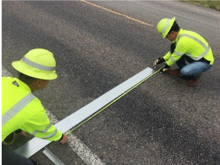
Figure 32. Marking the Position of the Metal Plates.
