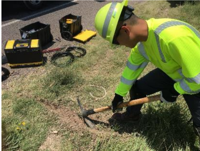
Figure 44. Digging a Trench.
