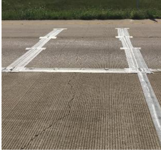
Figure 26. Portable WIM Installation on SH 130 in Travis County.
