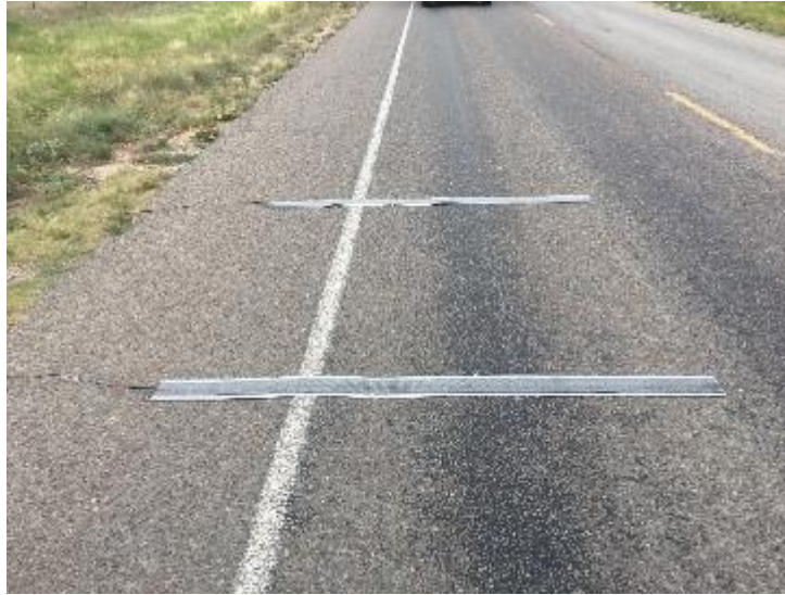
Figure 38. Imbedded Sensors on Top of Each Metal Plate.
