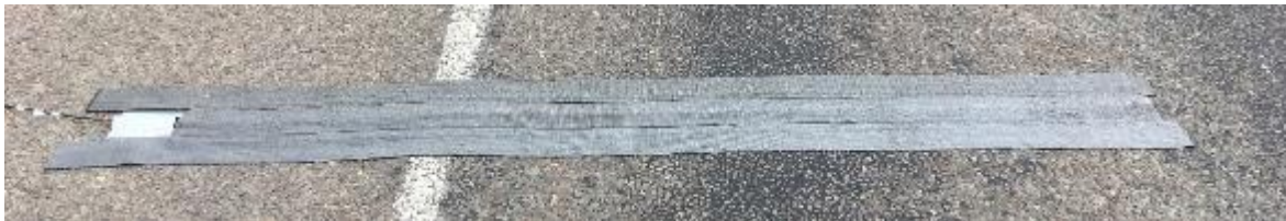
Figure 14. 4-Inch Road Tape Installed on the Road.
