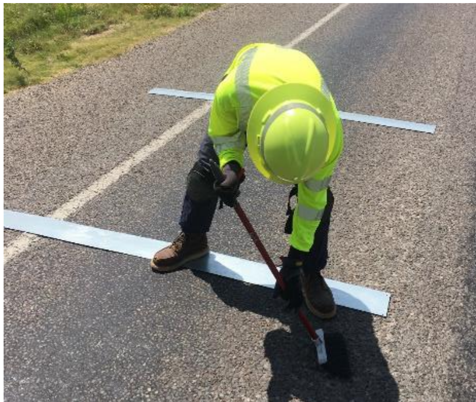
Figure 33. Cleaning the Marked Area.
