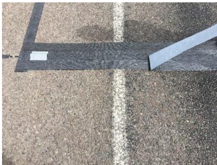
Figure 41. Applying 6-Inch Road Tape.
