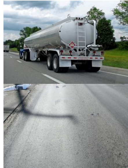
Figure 1. Surface Rutting.
