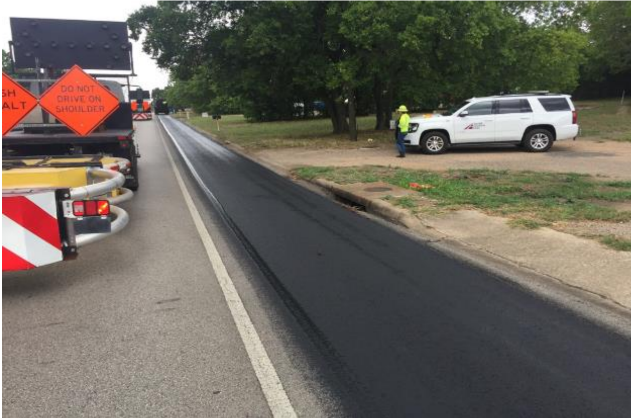
Figure 11. Fort Worth Test Section on Spur 102 near Keene, Texas.
