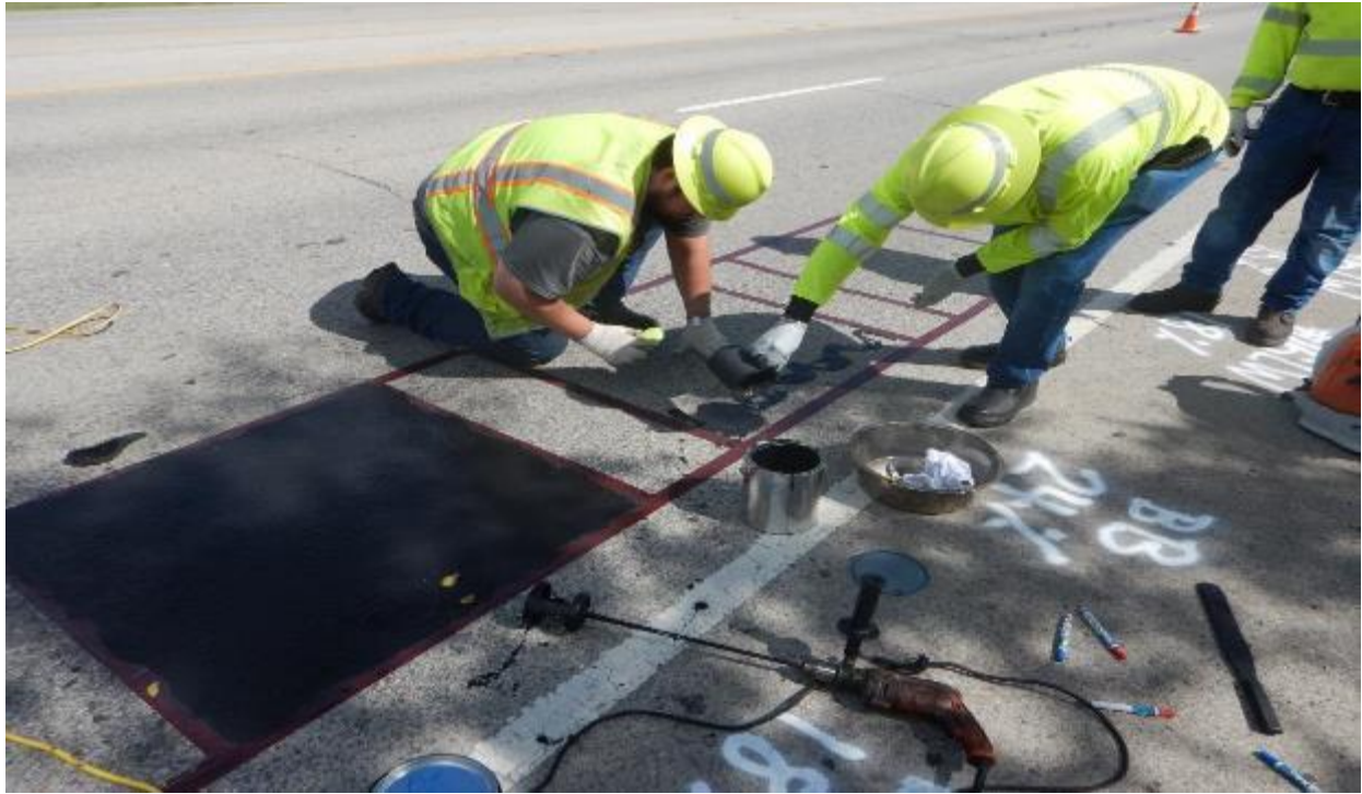
Figure 31. Application of UTSS on SH 21.
