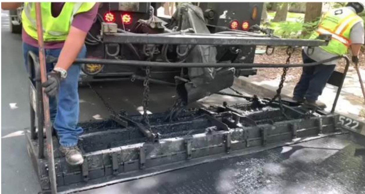
Figure 38. New Generation UTSS Application Equipment (Dec 2019 demo).
