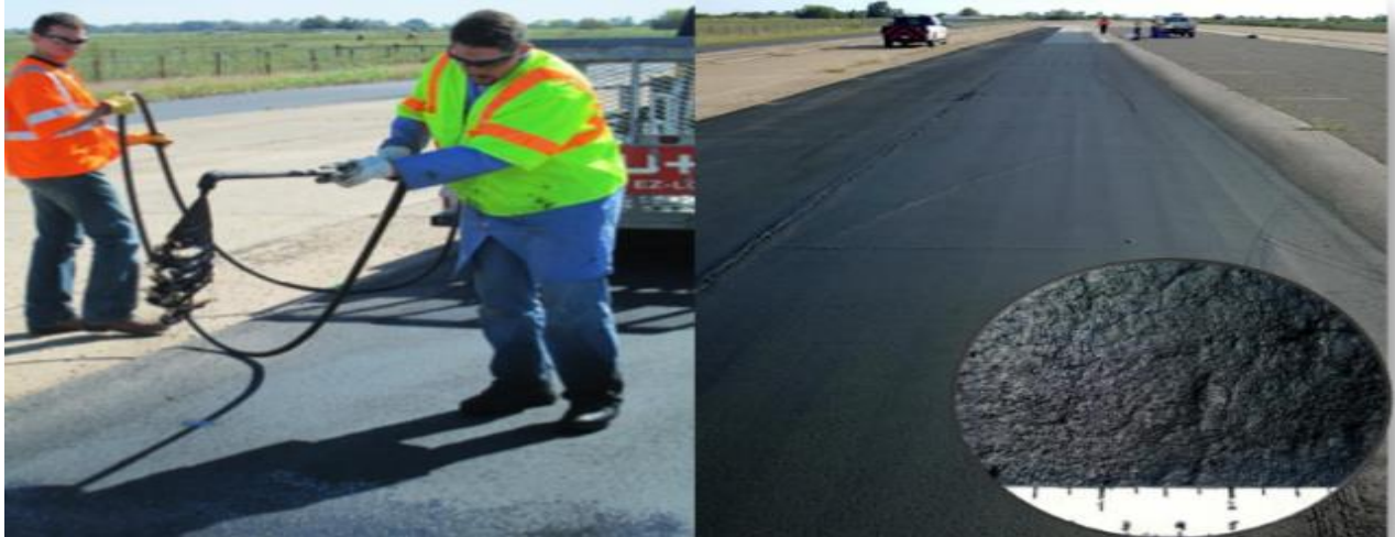
Figure 3. Application of UTSS (TTI Riverside Facility).
