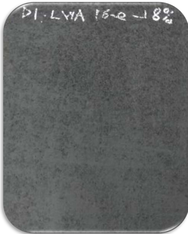
0.25gal/sy Light Weight UT Slurry on a Type D slab
