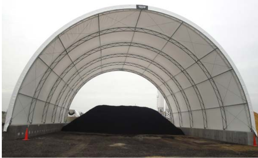
Figure 7. Covered RAS Storing Facility.
