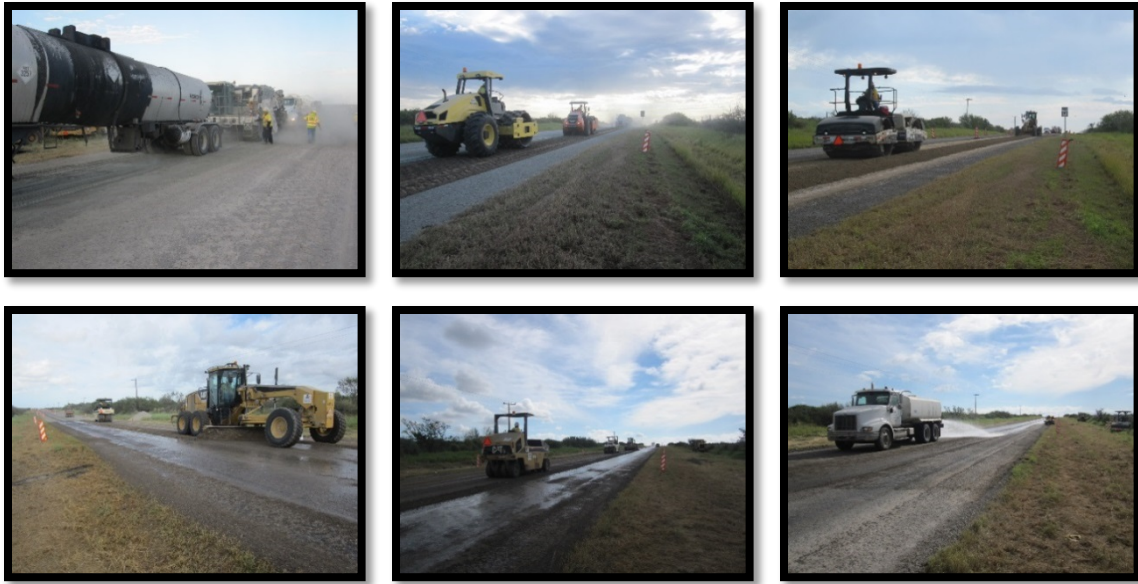
Figure 56. Typical Construction Sequence on SH 44.
