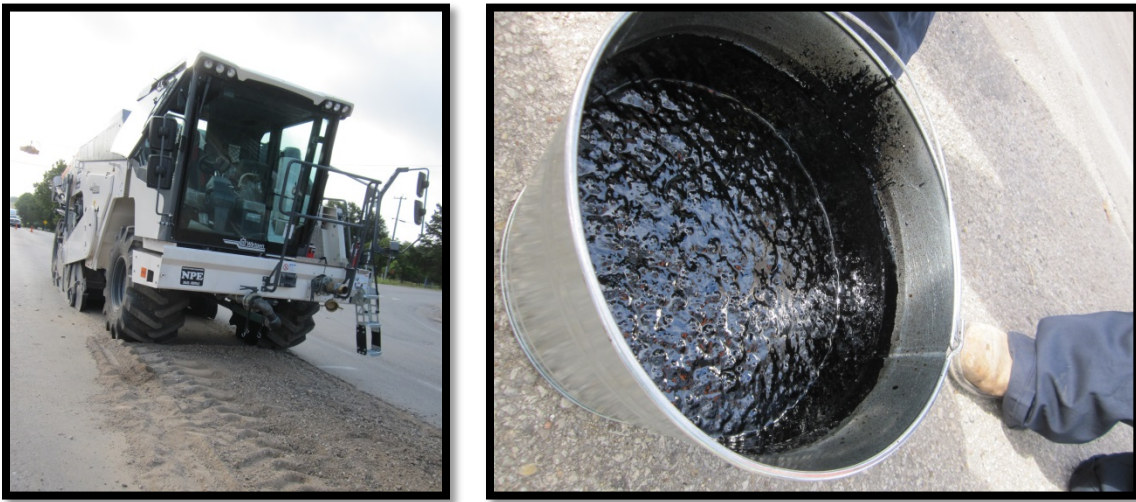
Figure 45. Checking Expansion Ratio and Half-Life of Foamed Asphalt on SH 7.
