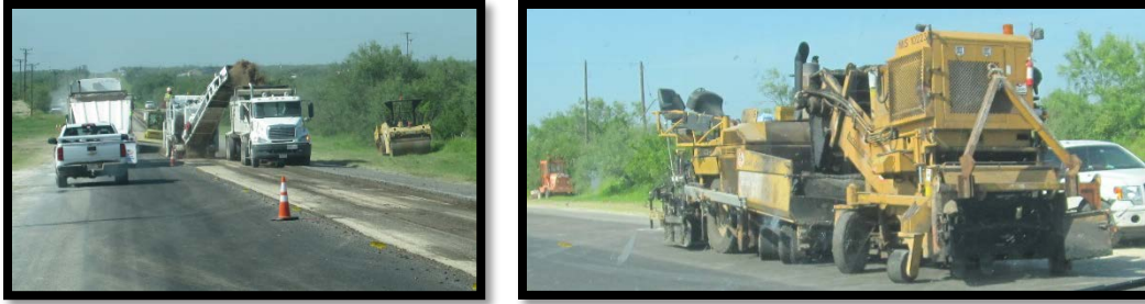
Figure 7. Mill and Inlay on SH 16.
