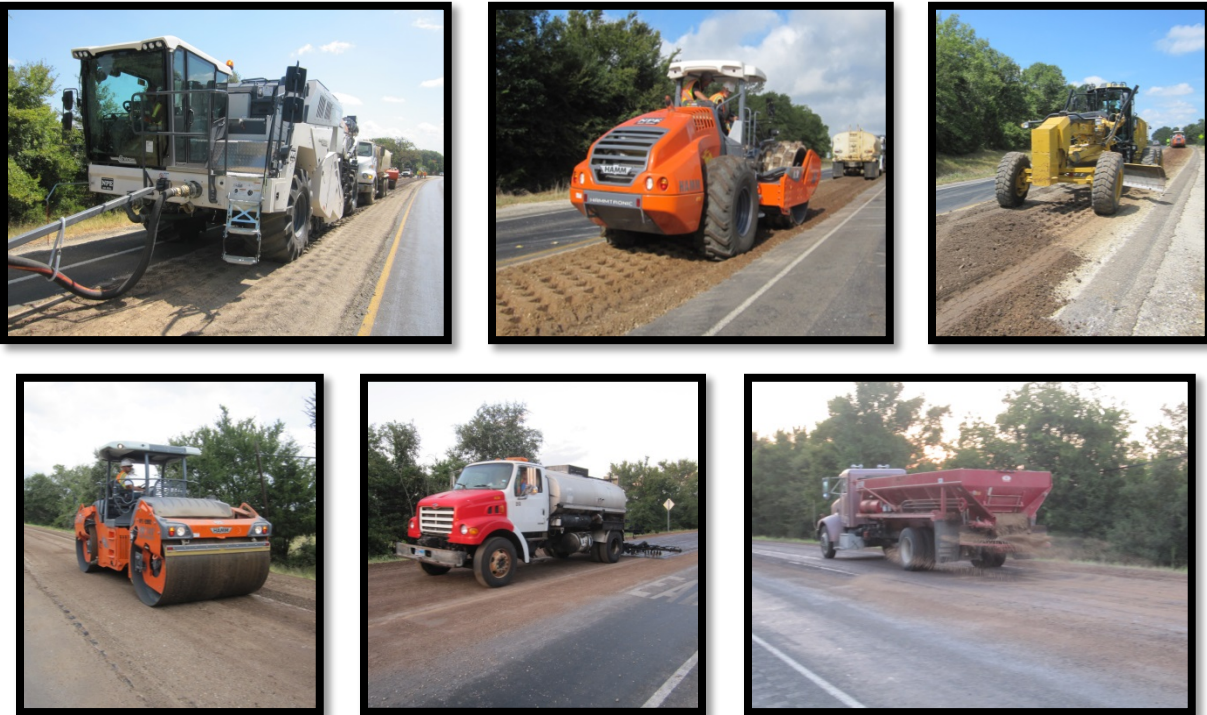
Figure 44. Typical Construction Sequence on SH 7.
