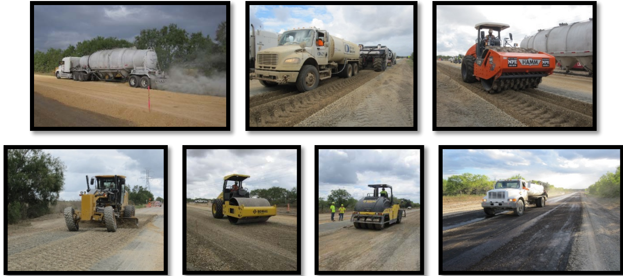
Figure 66. Typical Construction Sequence on FM 541.
