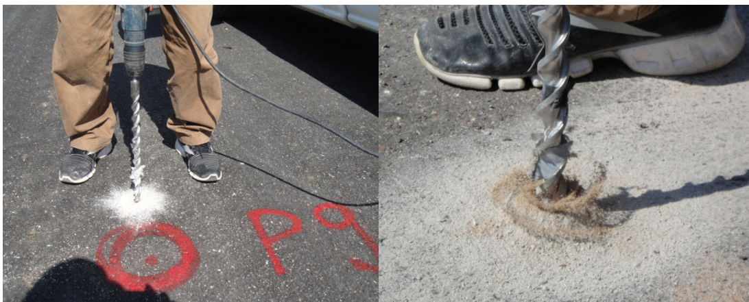
Figure 11. DCP Test after Placement of Stabilized Base.
