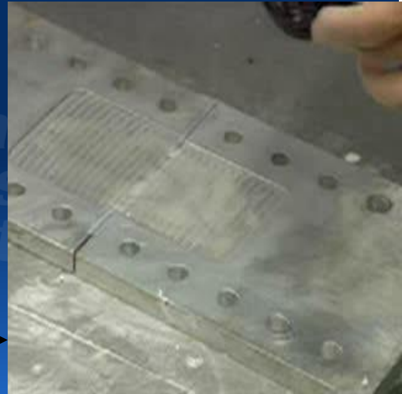
Reflection Cracking test
