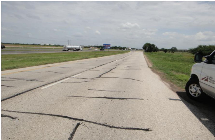
Figure 12. Existing Pavement Surface (Bryan-Fine SMA).
