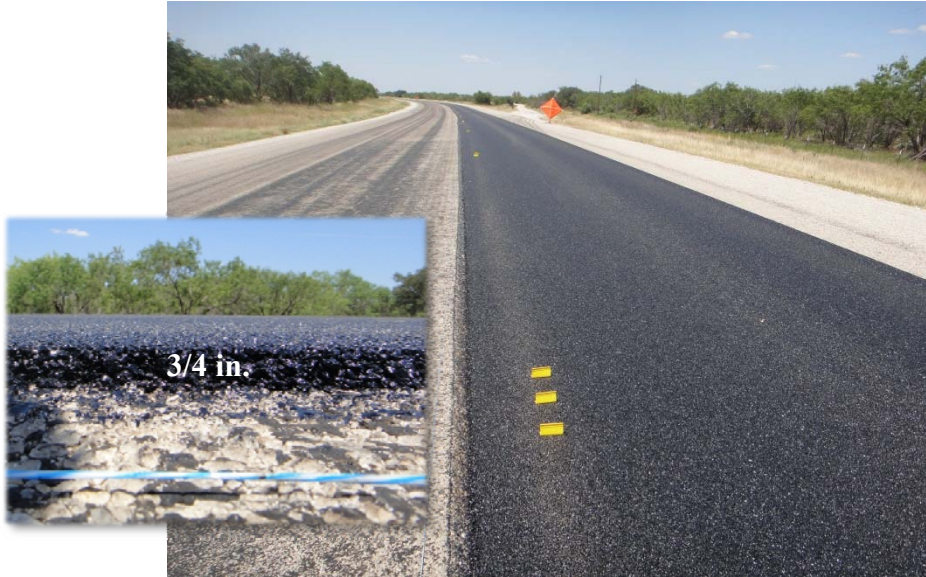
Figure 26. Project and Lift Thickness (Brownwood-Fine PFC).
