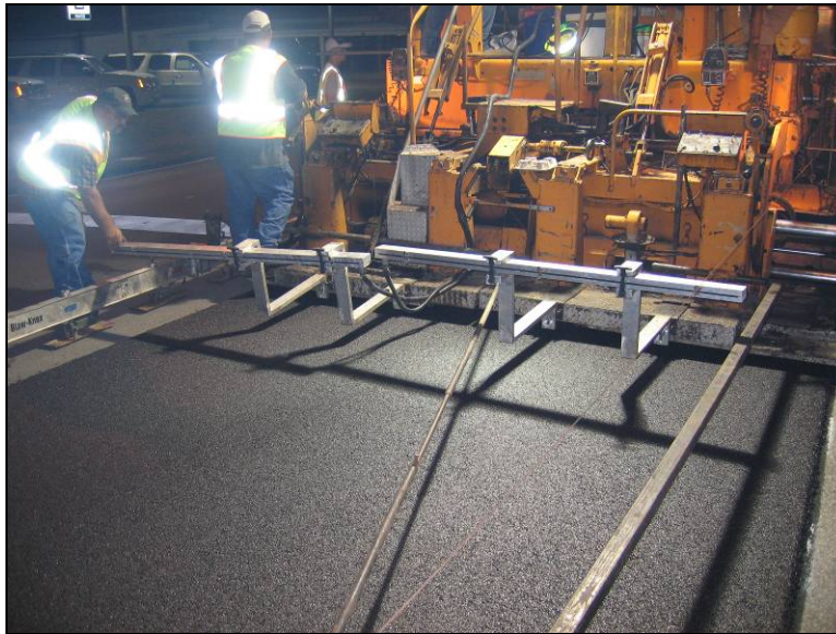
Figure 11. Pave-IR Collecting Thermal Profile on Business 59.
