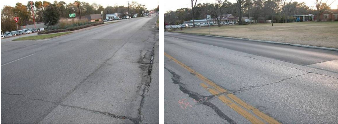
Figure 8. Location of Poor LTE on US 59 Prior to CAM Placement.
