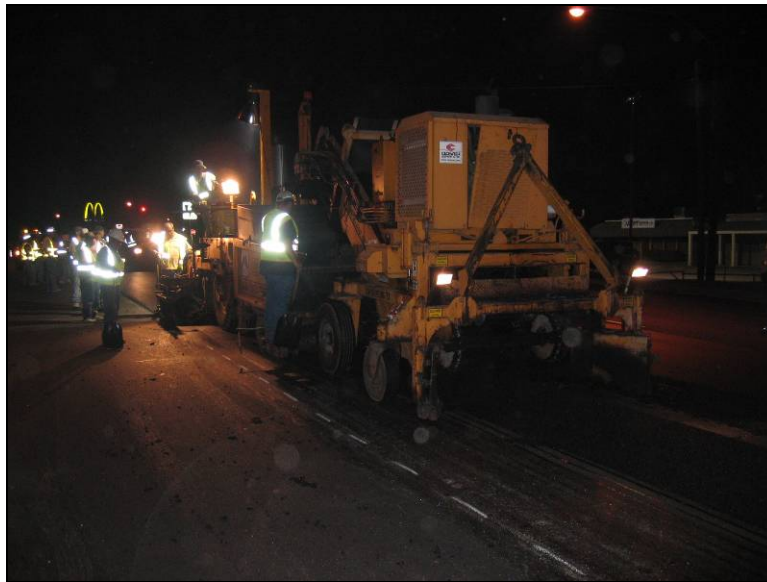
Figure 9. CAM Paving Operation on Business 59.
