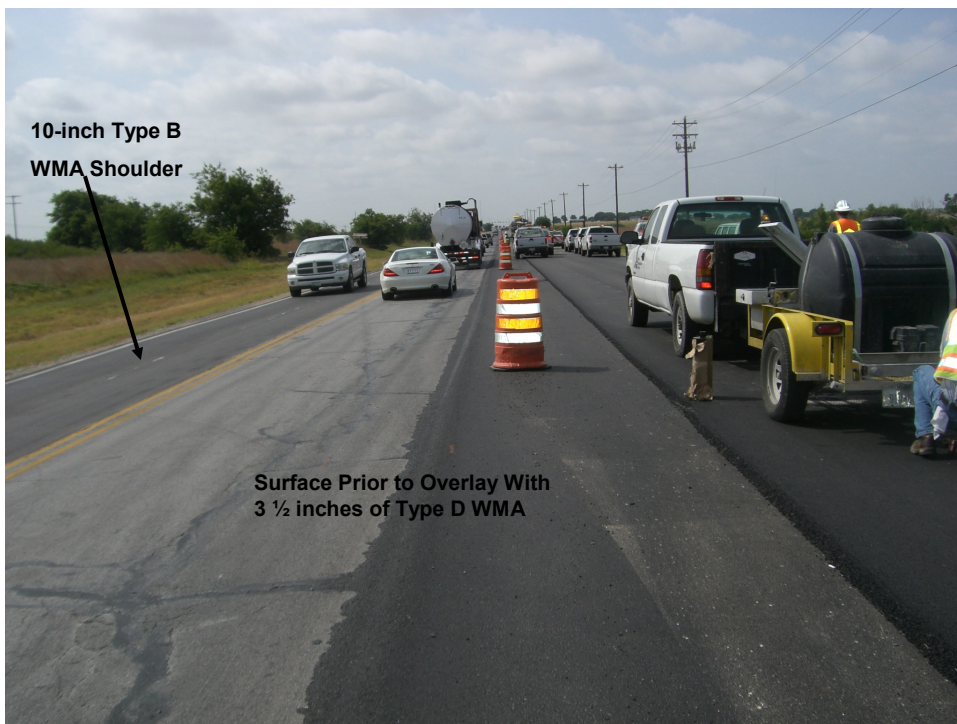
Figure 3.19. BU 287 Type B WMA Base Mix and Type D WMA Overlay.
