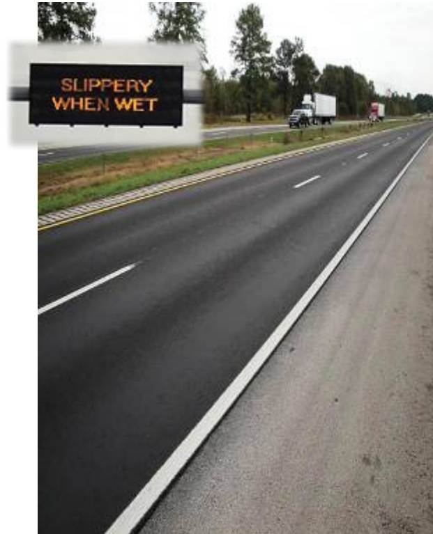
Figure 3.39. Severe Flushing (Atlanta-Fine SMA).
