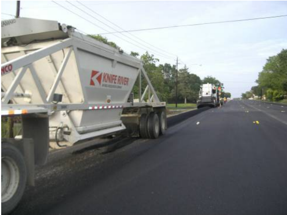
Figure 2.4. Foamed WMA Mixture Placement on SH 21 in Bryan.
