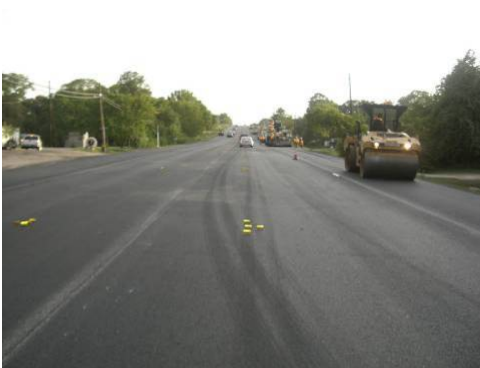
Figure 2.5. Foamed WMA Mixture Compaction on SH 21 in Bryan.
