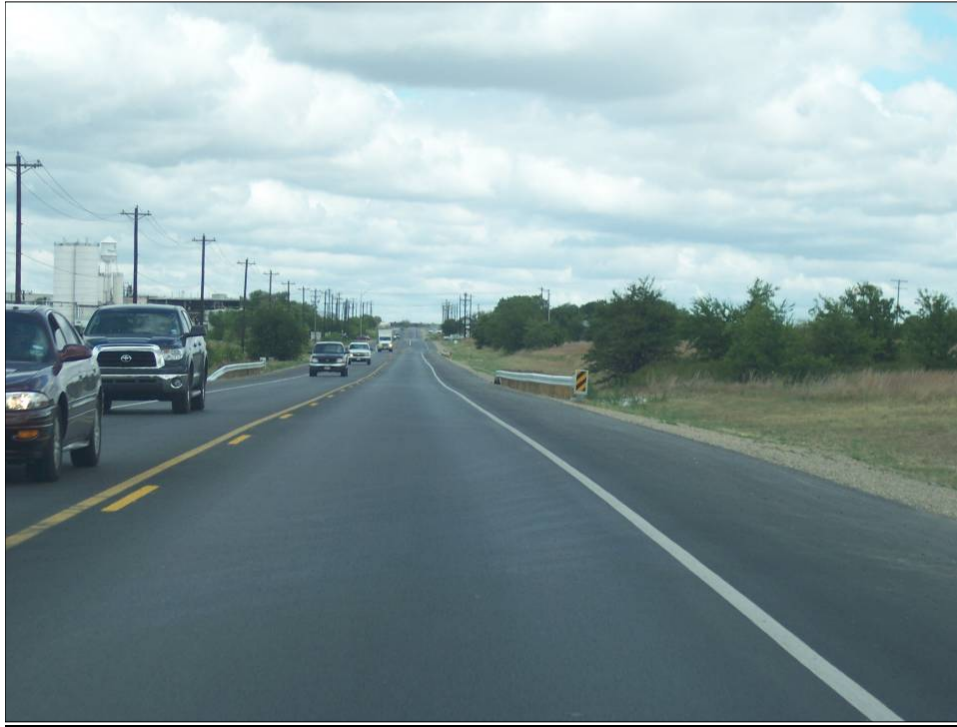
Figure 3.23. Fort Worth BU 287 WMA Project after One Year of Service.
