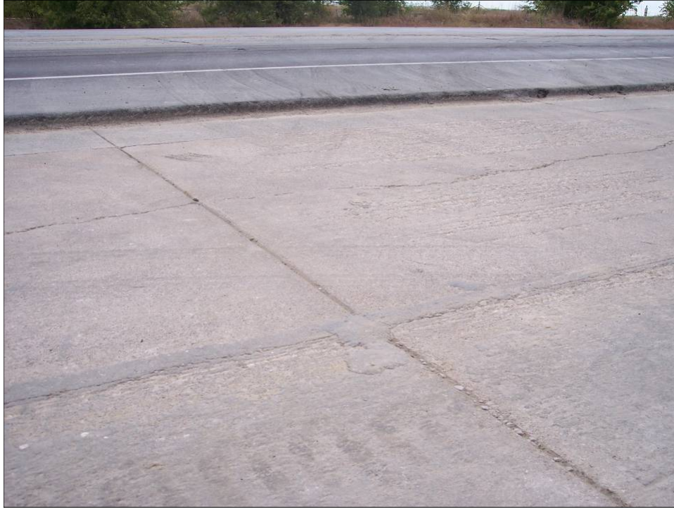
Figure 3.18. BU 287 Jointed Concrete Pavement prior to Type D WMA Overlay.
