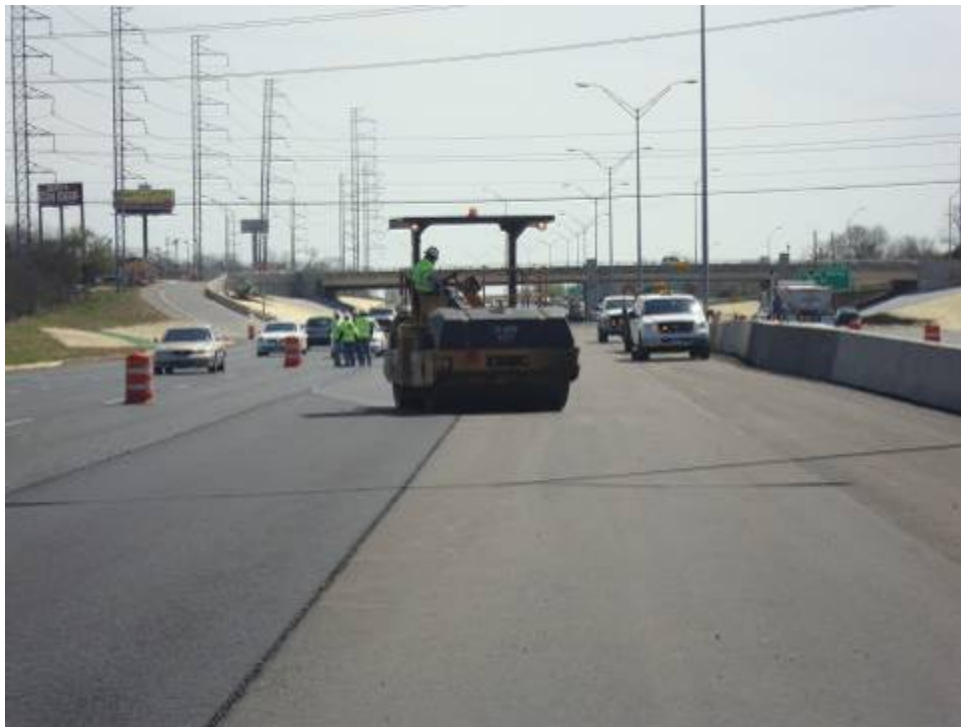
Figure 2.17. Compaction of WMA on IH 37 in San Antonio.
