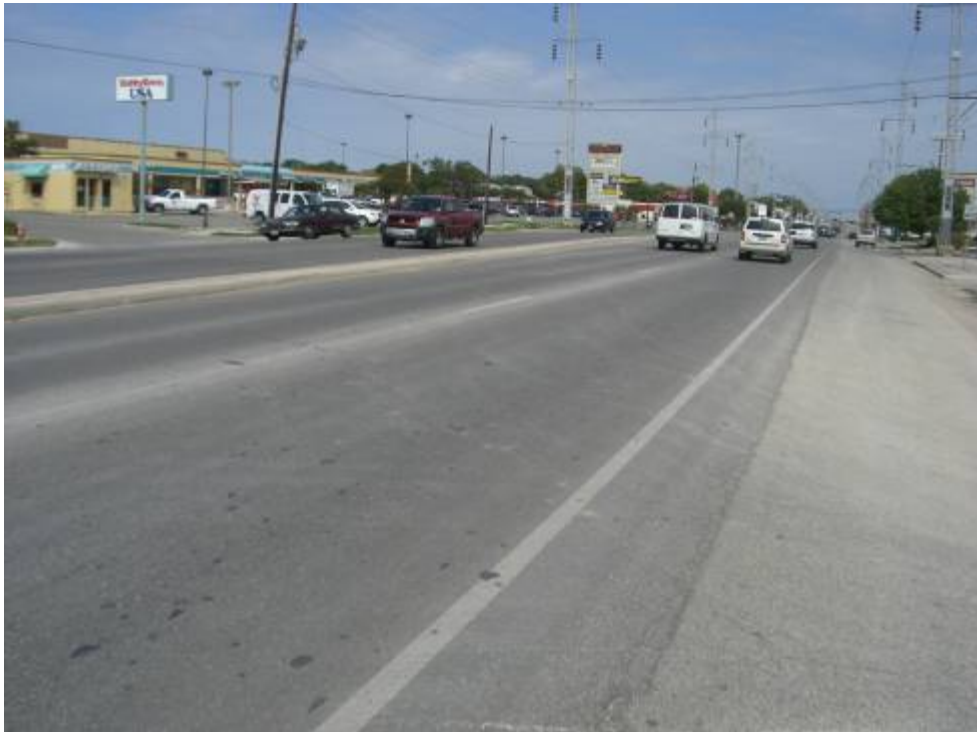
Figure 3.5. San Antonio Warm Mix Section after 3 Years of Service.
