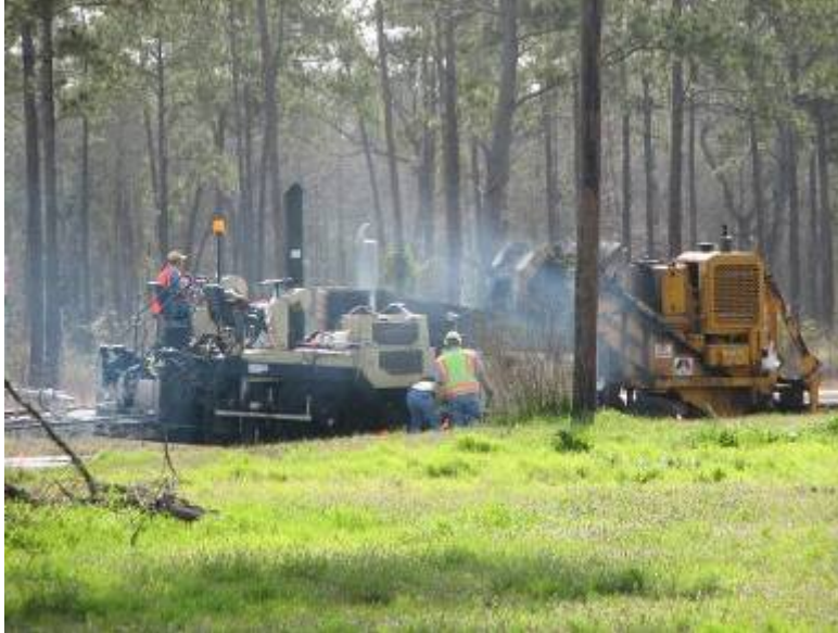
Figure 3.13. Construction of Lufkin WMA Field Trials.
