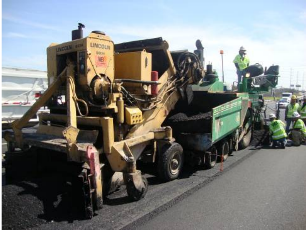
Figure 2.16. Placement of WMA on IH 37 in San Antonio.
