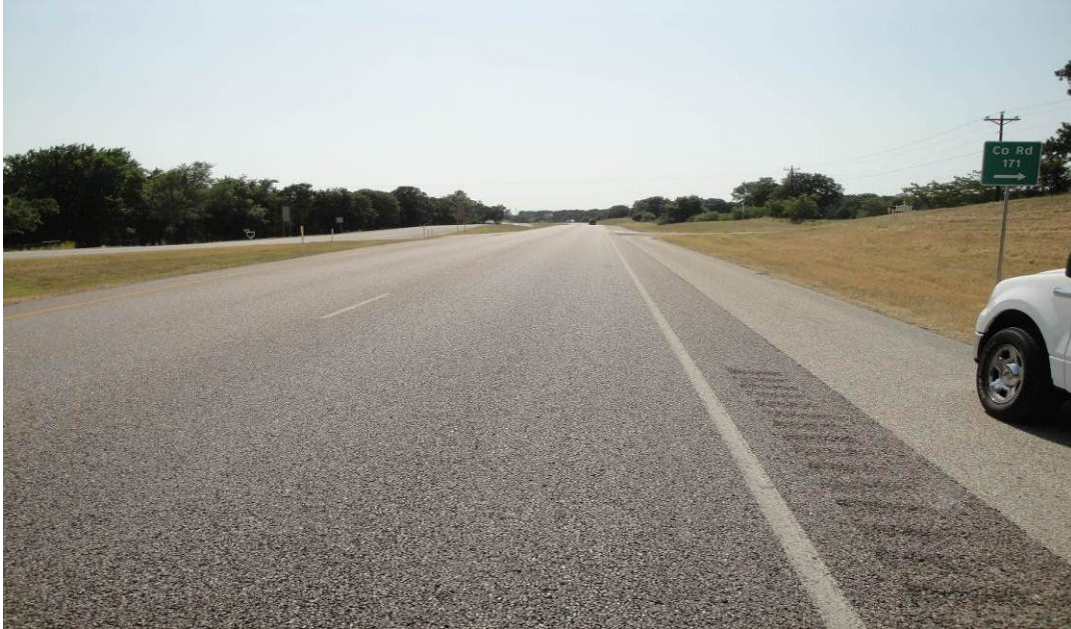
Figure 3-16. US 82 Overlay Section Overview.
