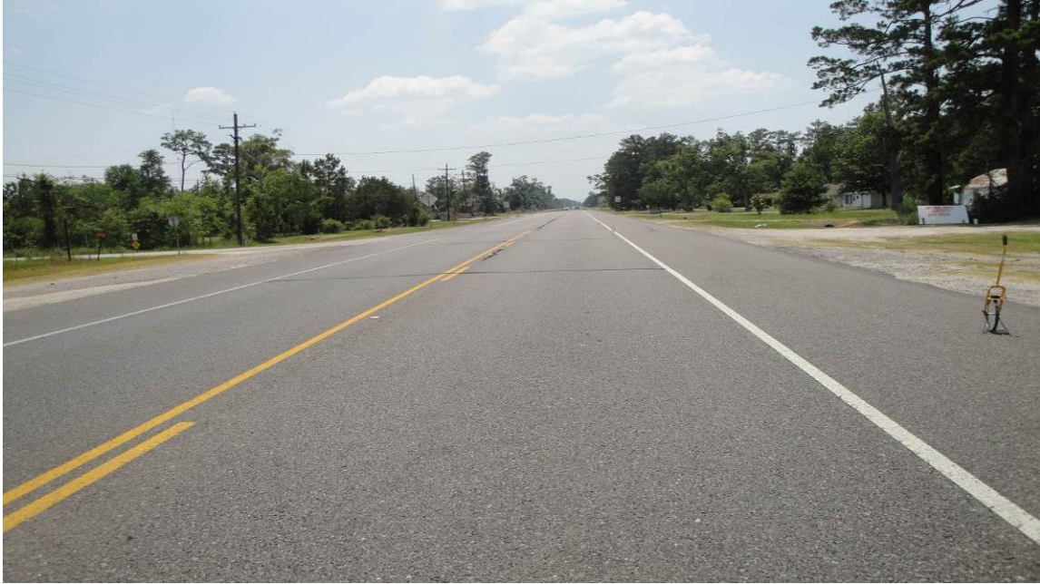
Figure 3-11. SH 12 Test Section Overview.
