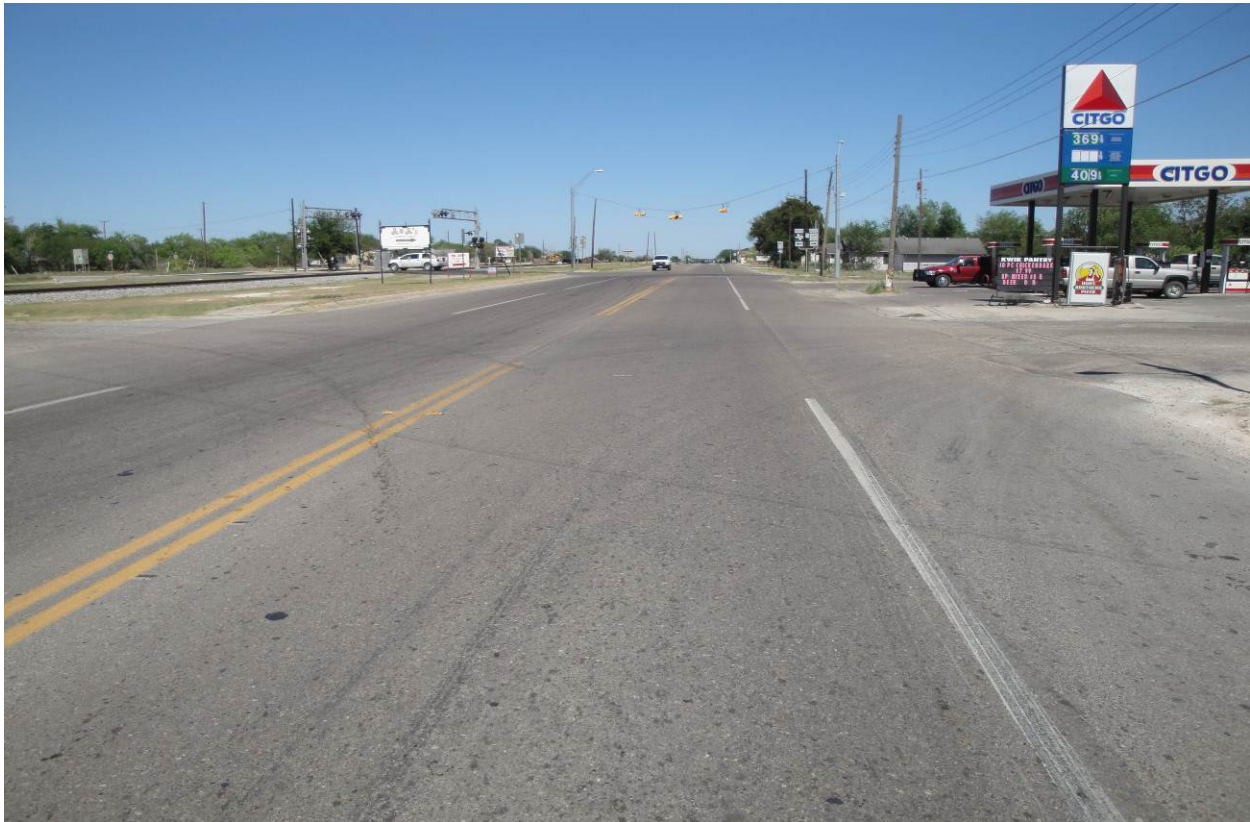
Figure 3-27. Overview of SH 359 Test Section.
