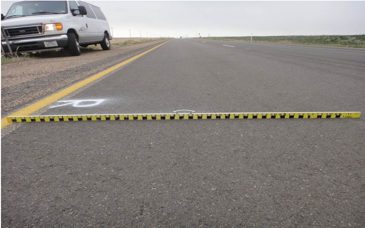
Figure 3-32. No Rutting in US 87 Test Sections, as of 5/30/2012.
