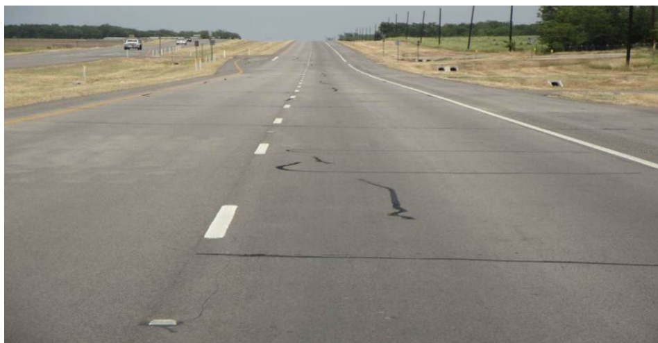
Figure 3-19. Overview of SH 24 Test Section.
