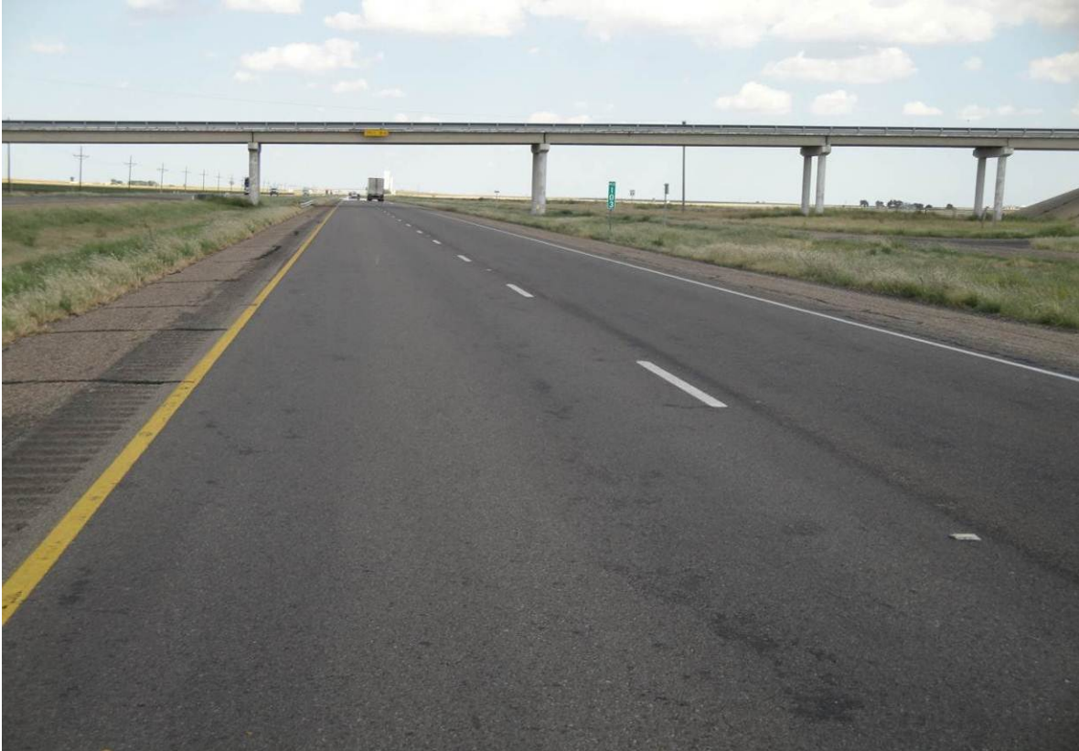
Figure 3-23. Overview of IH 40 Test Sections.
