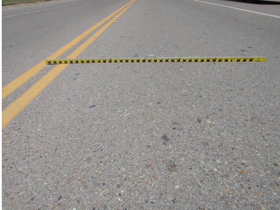
Figure 3-28. No Crack, No Rutting in SH 359 Test Section, as of 5/24/2012.
