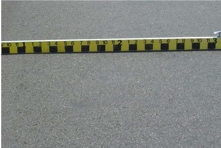
Figure 12. No Rut on the Main Traffic Lanes and Ramps.
