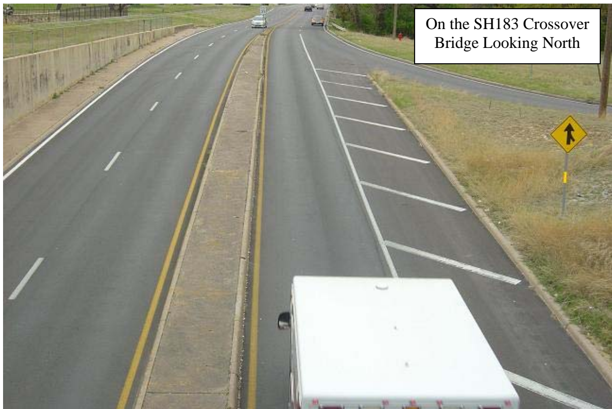
(14a). Overview of the Main Lanes between SH183 and the Naval Air Base Entrance.
