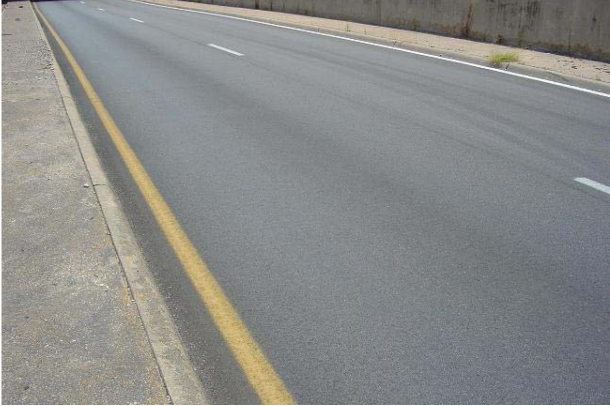
(14d). No Transverse Reflective Cracking: A Closer Look Figure 14. Field Observations of the Main Traffic Lanes.
