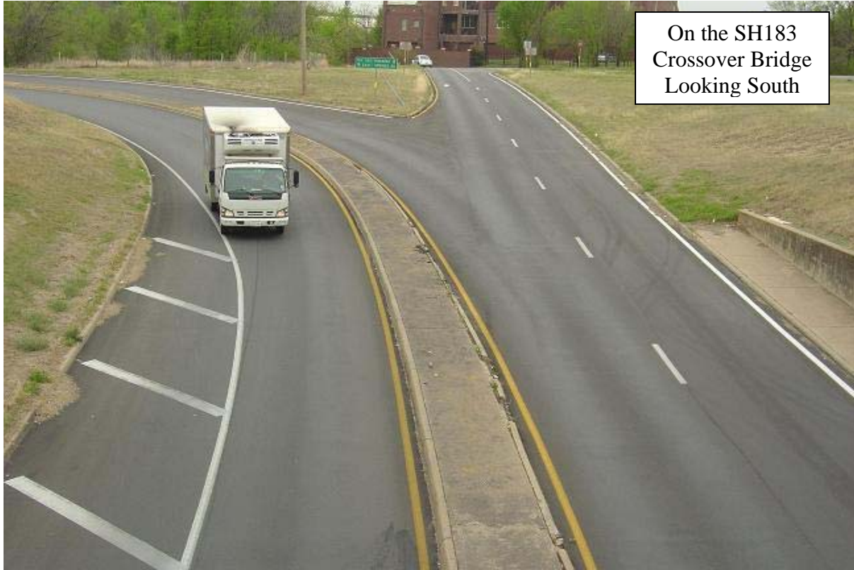
(14b). Overview of the Main Lanes South of SH183.
