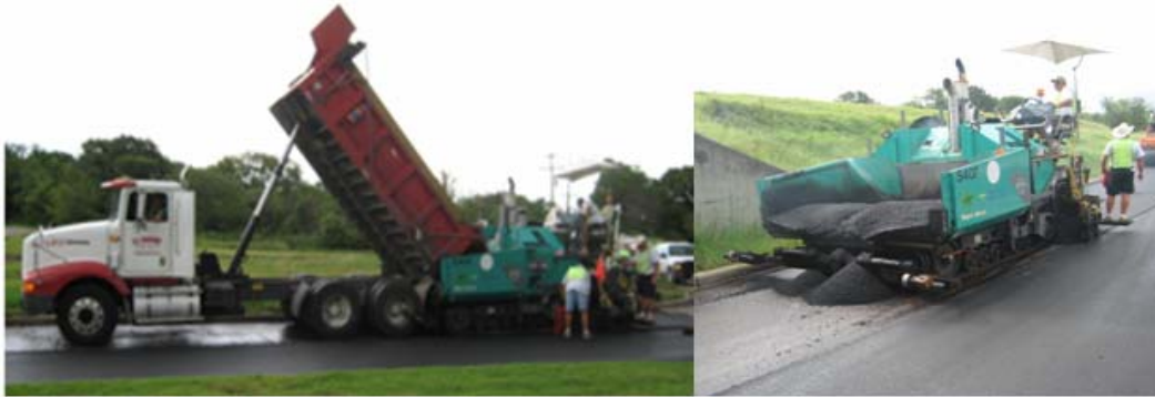
Figure 7. Paver Operation on the Pumphrey Drive, FTW.
