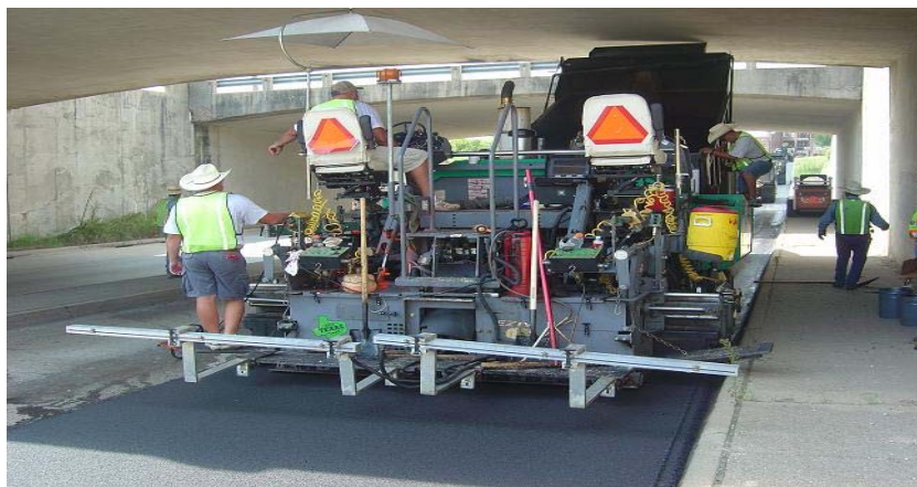
Figure 8. Temperature Measurement Using the Infra-Red Bar during Construction.
