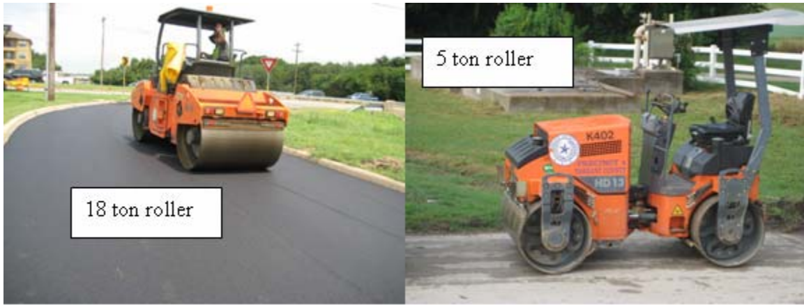
Figure 10. Rolling Compaction – Tarrant County 18- and 5-Ton Rollers.
