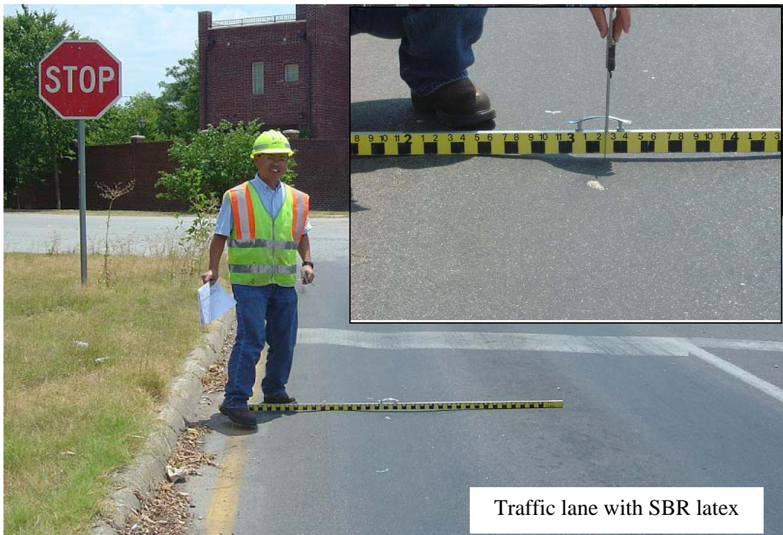
Figure 13. Observed Rut at the Stop Sign at Roaring Springs Road.
