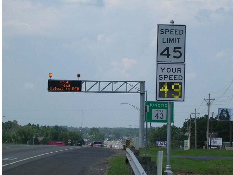
Figure 10. Overhead Electronic Matrix Sign.
