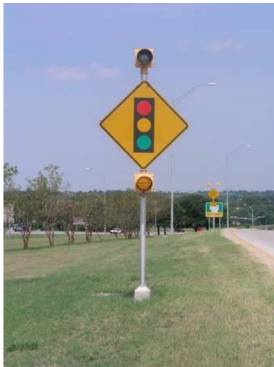
Figure 7. Signal Ahead Sign (W3-3) with Beacons.
