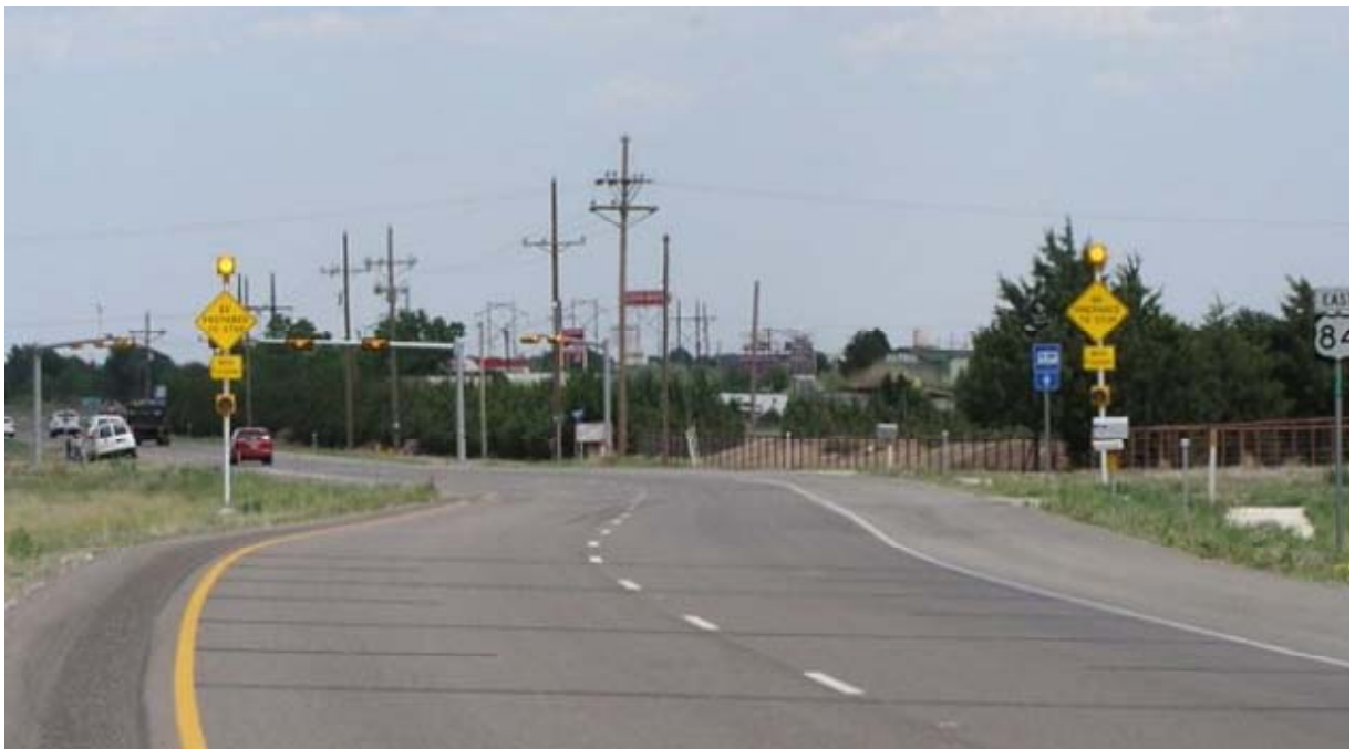
Figure 4. AWEGS Signs on a Two-Lane Approach.
