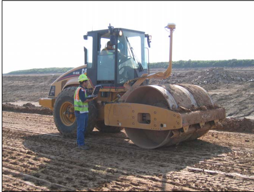
Figure 2.7 Collecting Roller Drum Displacement Data on SH 130.
