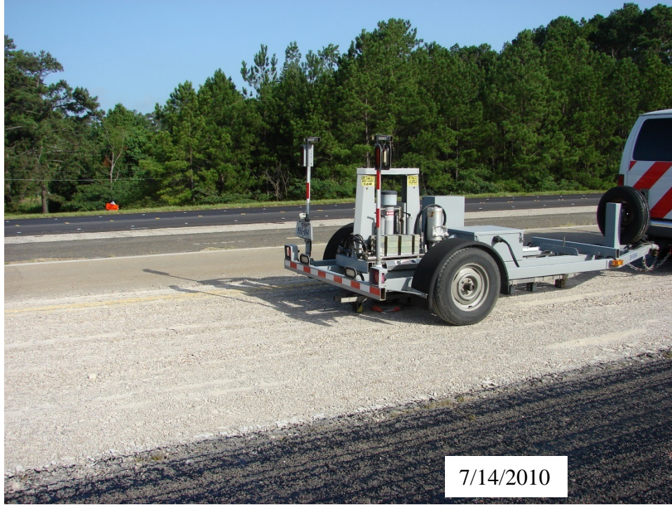
Figure 23. FWD Testing on Top of Rubblized Concrete (Rubble).
