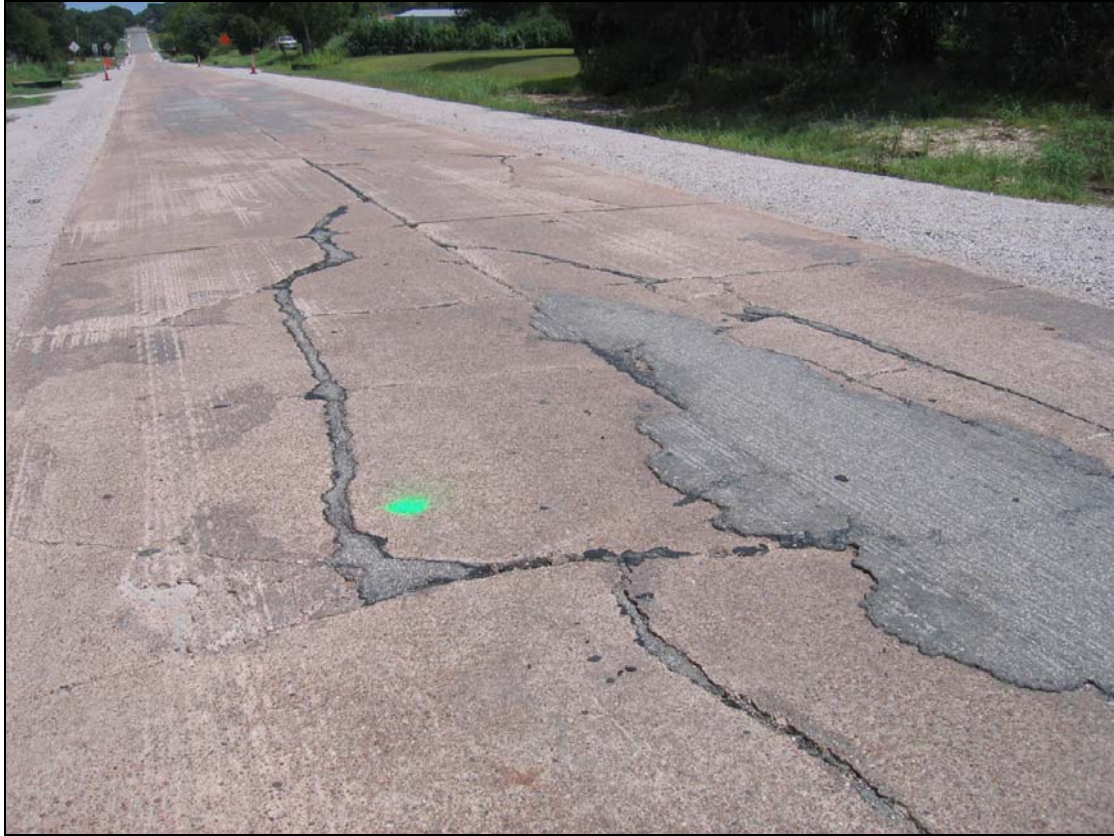
Figure 2.10. Existing JCP at Station 214.
