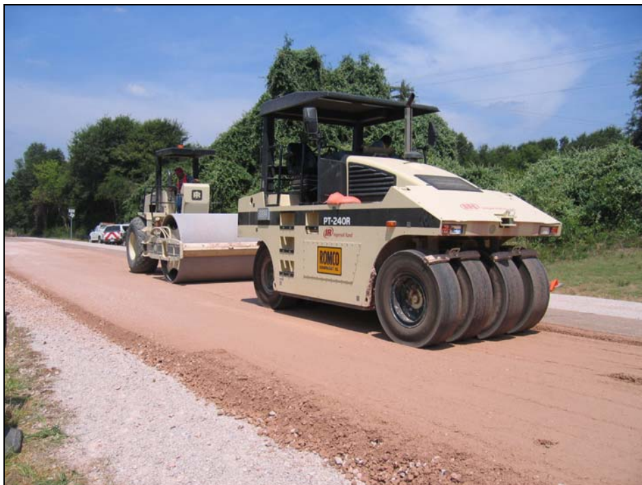
Figure 2.13. Compacting Base with Pneumatic and Steel Wheel Rollers.
