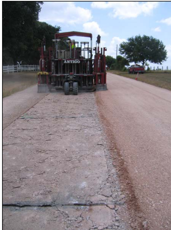
Figure 2.5. Modified Break Pattern with Type II Rubblization.
