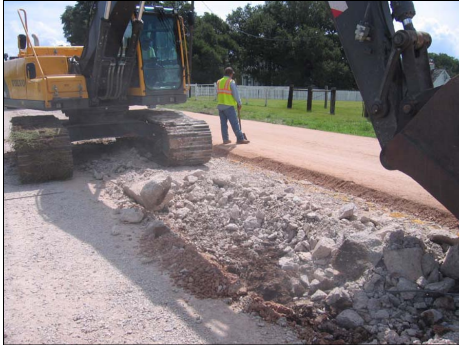
Figure 2.8. Test Pit with Type I Equipment.
