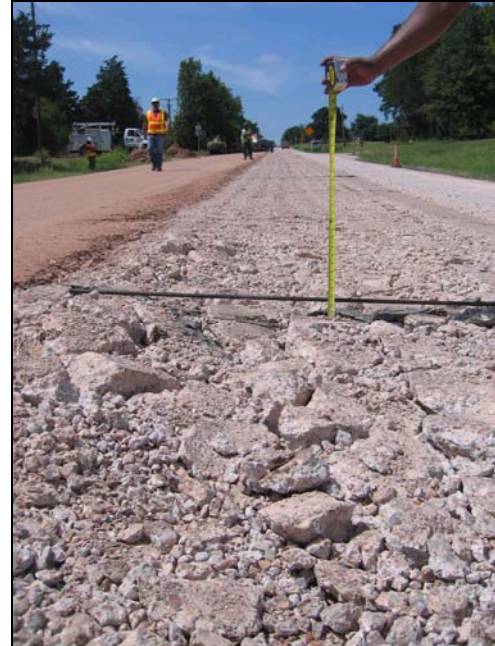
Figure 2.9. Example Location Requiring Full-Depth Repair with Type I Rubblization.
