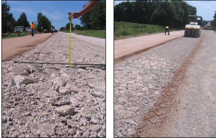
Figure 4.2. Poor Break Patterns Observed at Areas of Instability from Type I (Left) and Type II (Right) Equipment.
