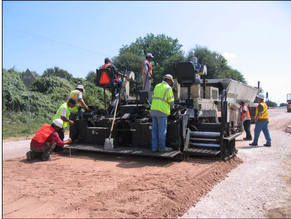
Figure 2.12. Placing Base with Paver.
