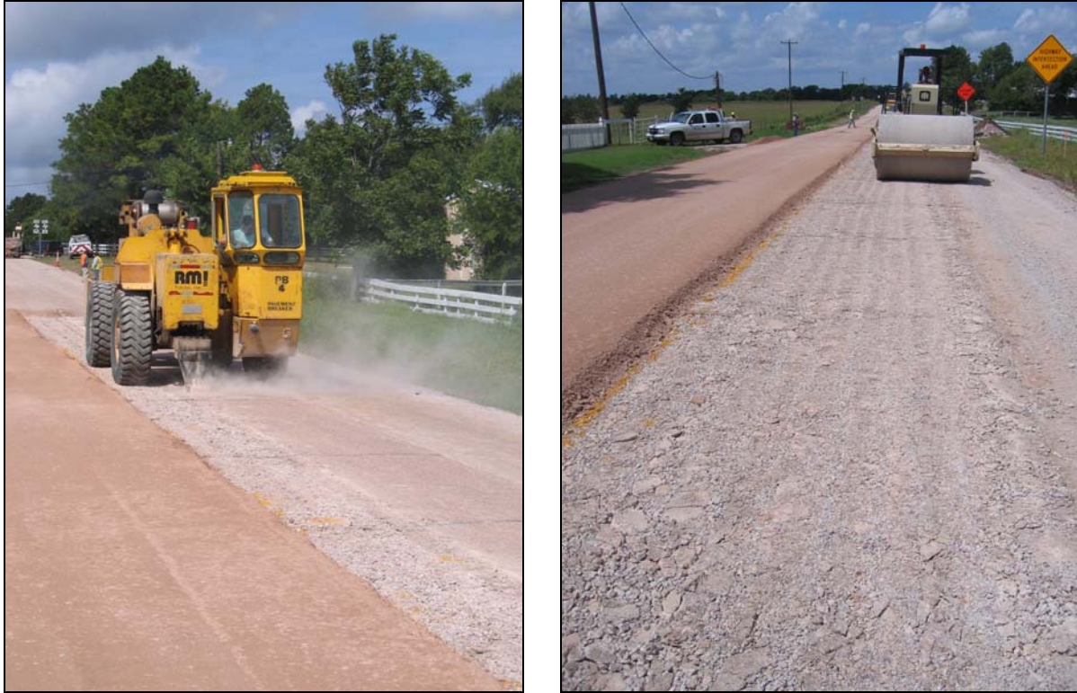
Figure 2.7. Type I Rubblization in Progress and Completed Section.
