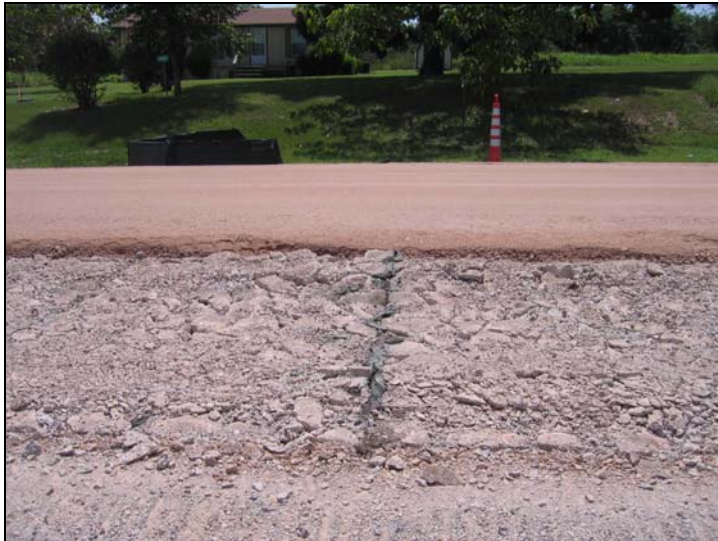
Figure 2.9. Example Location Requiring Full-Depth Repair with Type I Rubblization.
