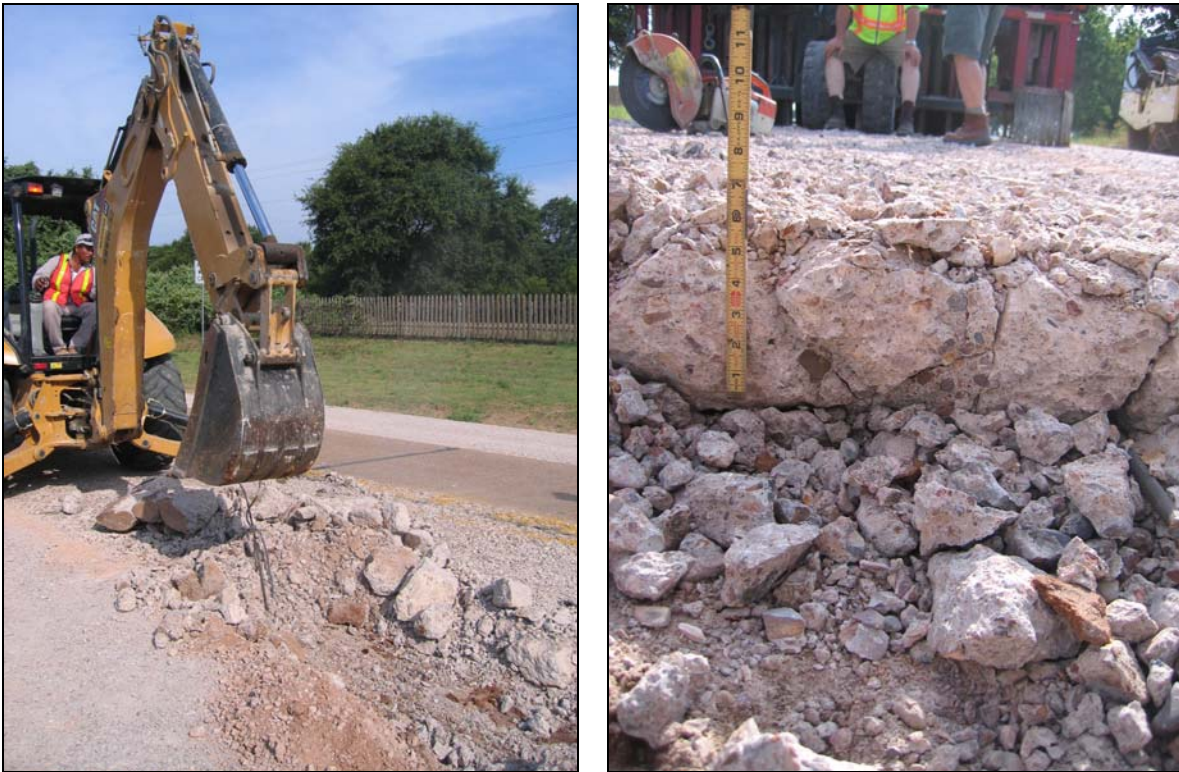
Figure 2.2. Surface and Side View of Test Pit with Type II Rubblization.
