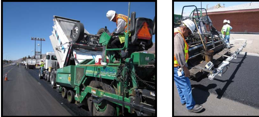
Figure 28. Paving TY C Mix on Dyer Street.
