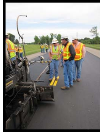
Figure 22. Pave-IR Collecting Project Data on SH 8.
