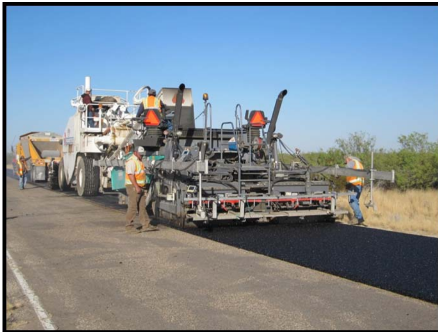
Figure 16. Paving Operation on Pecos Test Sites.
