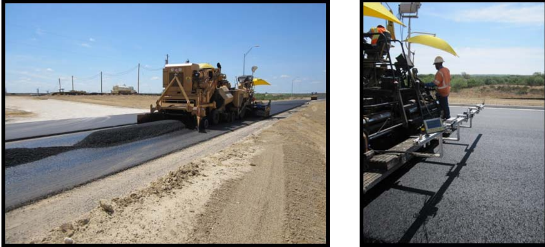
Figure 33. Paving TY C Mix on SL 20.
