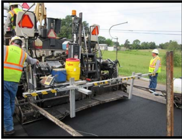
Figure 22. Pave-IR Collecting Project Data on SH 8.
