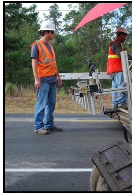
Figure 41. Paving on FM 2854 with Pave-IR Data Being Collected.
