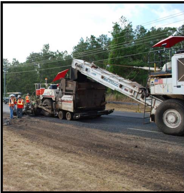
Figure 41. Paving on FM 2854 with Pave-IR Data Being Collected.
