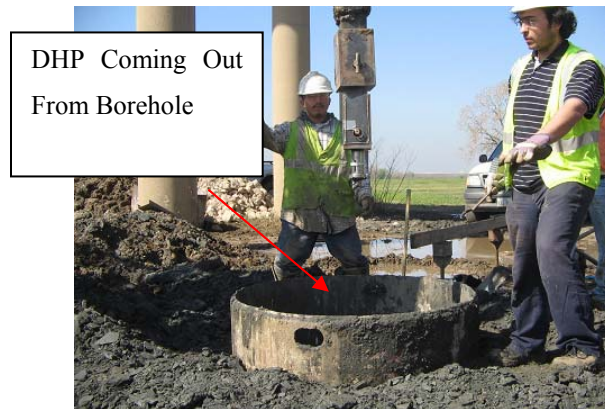
Figure 3.25 DHP Taken Out of the borehole
