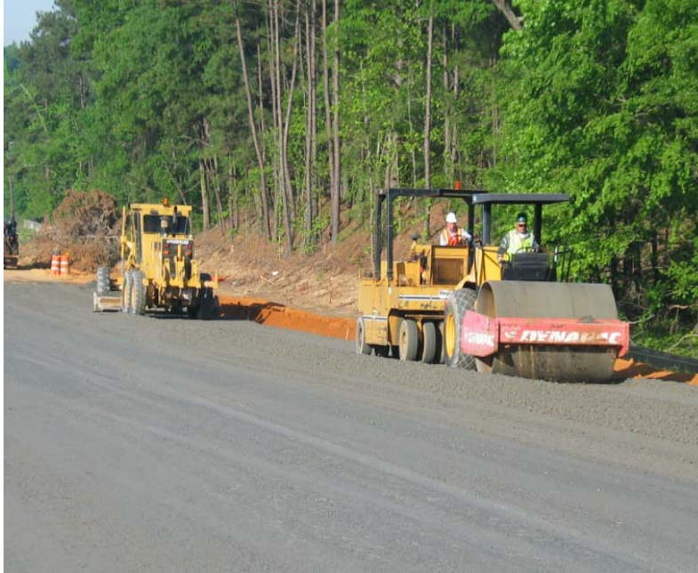
Figure 2. Compaction Sequence on SH 31.
