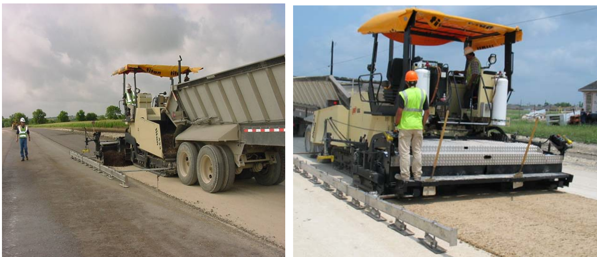
Figure 8. Base Paver Operations in the Waco District.
