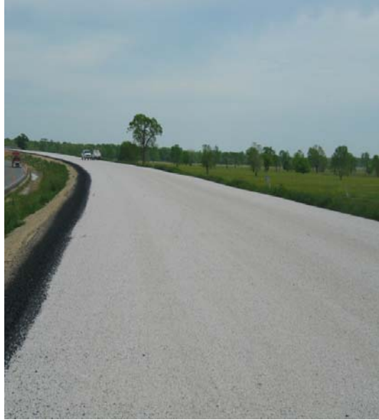
a) underseal prior to HMA placement
