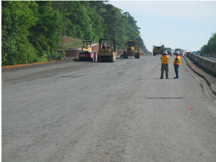
Figure 1. Granite Mountain Base Being Placed on SH 31.
