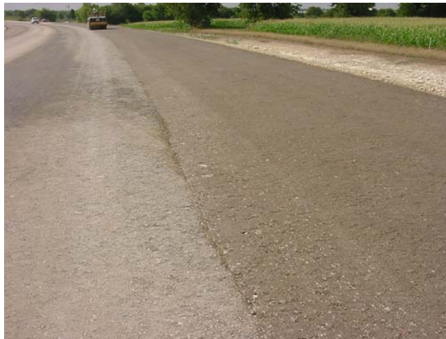
Figure 9. Smooth Ride and Excellent Joints in Paver-Placed Base Layer.
