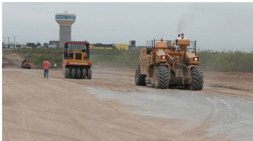
Figure 2.6. Pneumatic Roller Used to Prepare the Surface for Lime Placement.
