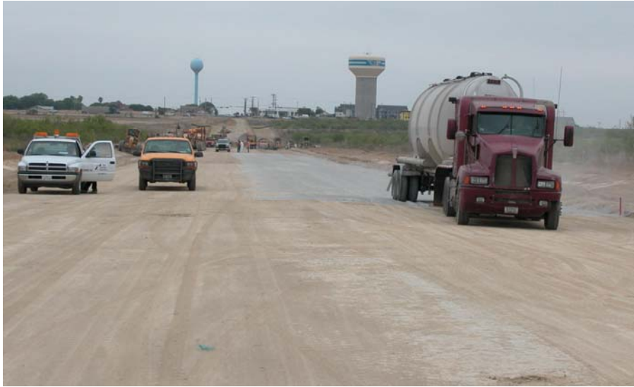
Figure 2.3. GGBFS Being Spread along the Project in Eagle Pass.
