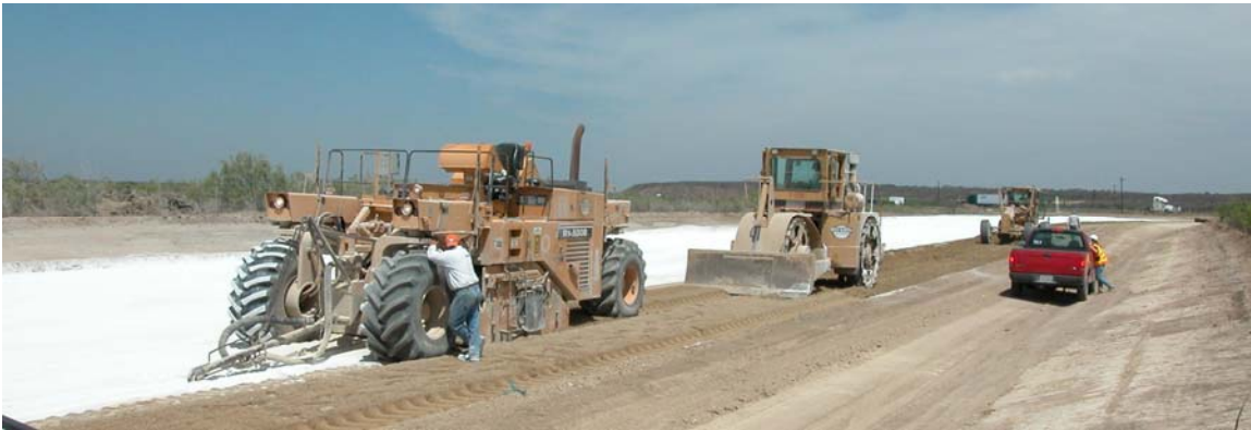
Figure 2.9. Progress Halted by CMI Waiting on a Water Truck.
