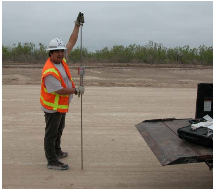
Figure 2.2. Ramon Rodriguez Collecting DCP Data on the Second Street Project.
