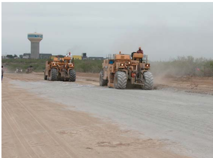
Figure 2.4. CMI's Used to Mix the GGBFS into the Subgrade.
