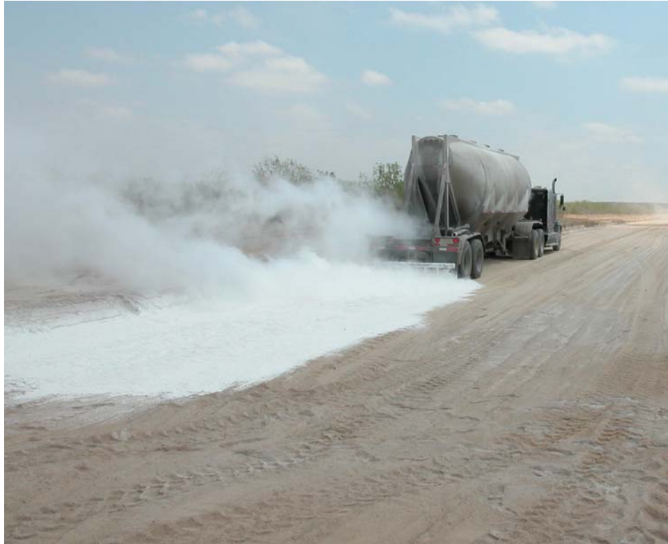
Figure 2.7. Application of the Lime to the Subgrade Following GGBFS Placement.
