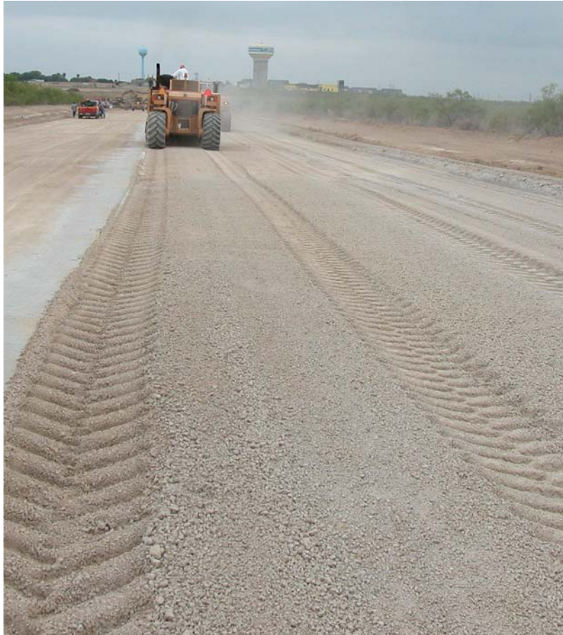
Figure 2.5. The CMIs Efficiently Mixed the GGBFS into the Subgrade.
