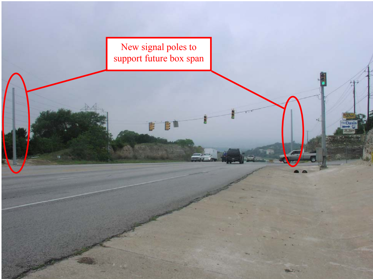
Figure 10. Westbound Approach to RM 620/Comanche Trail Intersection.
