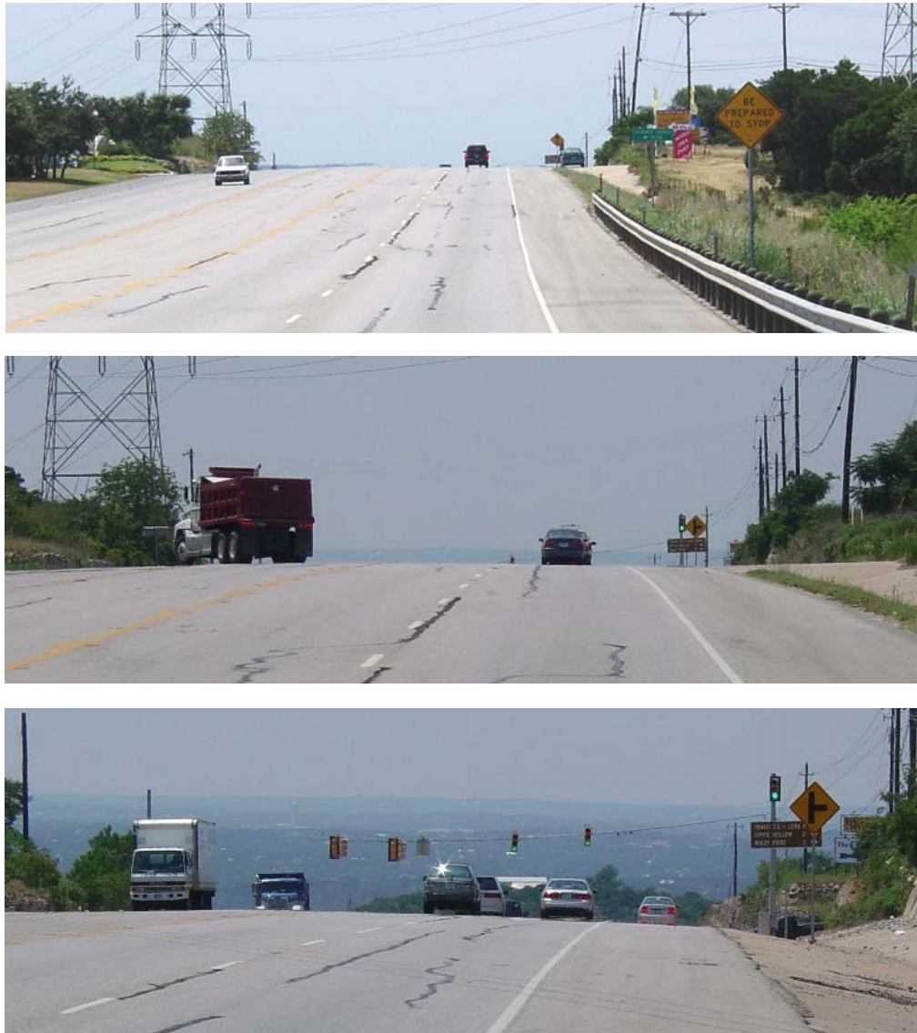
Figure 7. Westbound RM 620 Approaching Comanche Trail.
