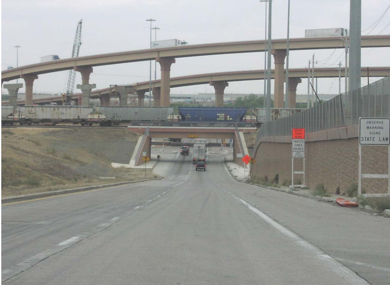
Figure 19. Westbound Loop 20 Approaching the Union Pacific RR Bridge and I-35.
