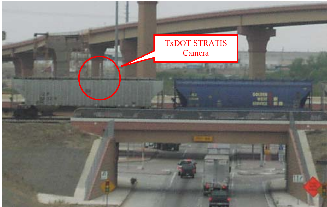
Figure 21. TxDOT STRATIS Camera and Pole Above UP Train and Tracks.
