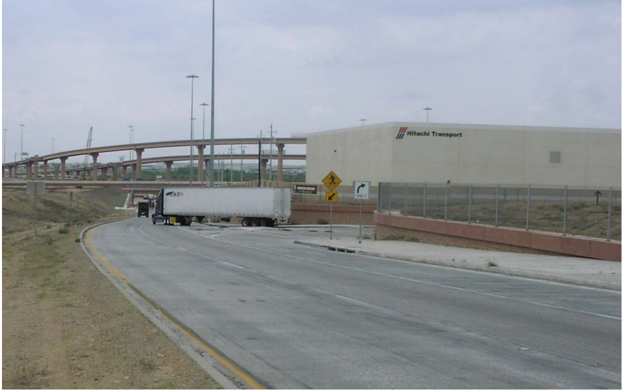
Figure 20. Warehousing Building North of Loop 20 Westbound Approaching I-35.
