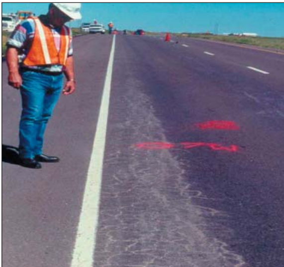
Figure 1. Distressed Flexible Pavement.
