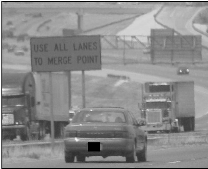
Figure 4. 'Use All Lanes to Merge Point' Sign for Three to Two-Lane Closure Scenario.
