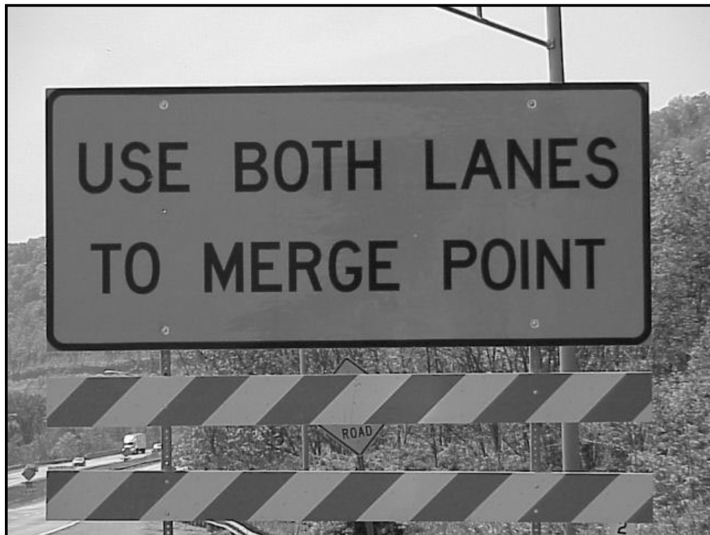
Figure 5. 'Use Both Lanes to Merge Point' Sign for Two to One-Lane Closure Scenario.
