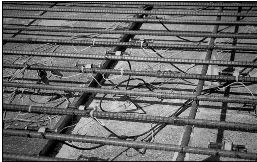
Figure 3.3 Concrete Strain Gages Installed before Paving.
