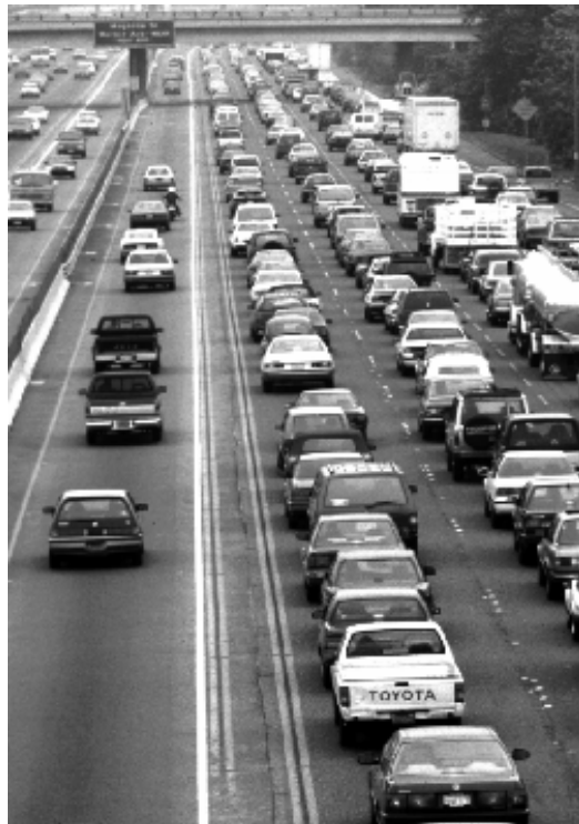
Figure 7. IH-405 Buffer-Separated Concurrent-Flow HOV Lane in Orange County, California (2).
