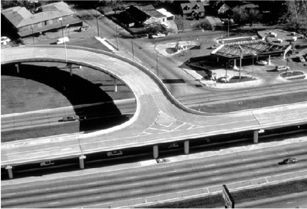
Figure 10. IH-45 Gulf Freeway T Ramp in Houston, Texas (2).
