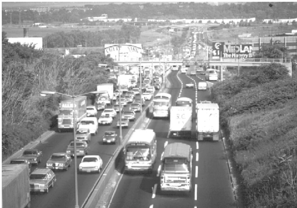
Figure 9. IH-495 Union City, New Jersey, Contraflow Lane (2).
