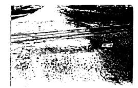
Figure 2. Typical Ratings for Edge Ravelling
