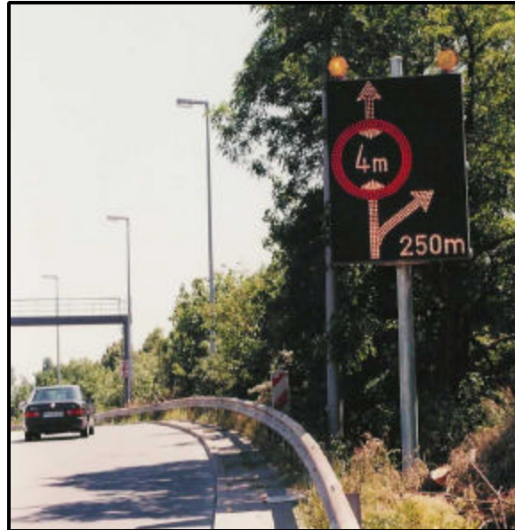
Figure 2-18. Small Roadside VMS on Autobahn 100 in Germany. 39
