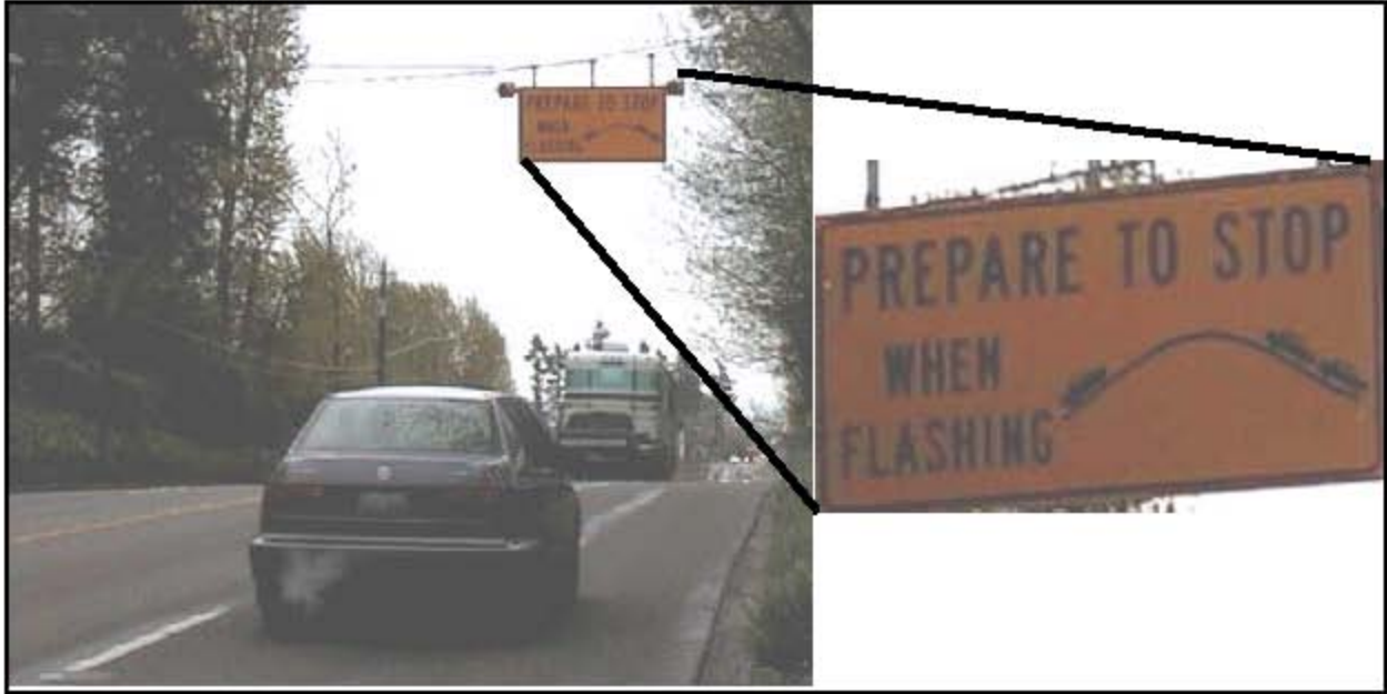
Figure 2-46. Picture of King County Queue Warning Sign near Elementary School. 91
