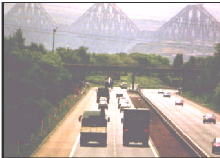
Figure 2-33. COMPANION System in Scotland. 51
