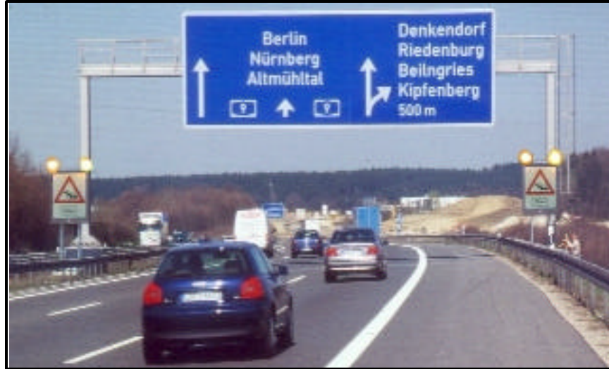
Figure 2-16. Mobile Traffic Jam Warning System on Autobahn 9. 38
