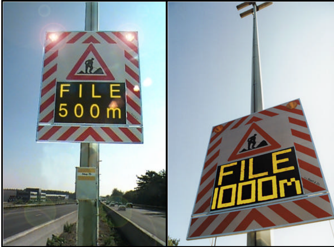
Figure 2-7. Activated VMS Panels in the Queue Detection and Warning System. 27
