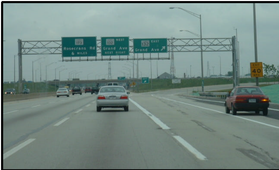
Figure 2-40. Picture Showing the Tri-State Tollway Bottleneck Improvement Conversion to a 2-lane Exit at Grand Avenue. 75
