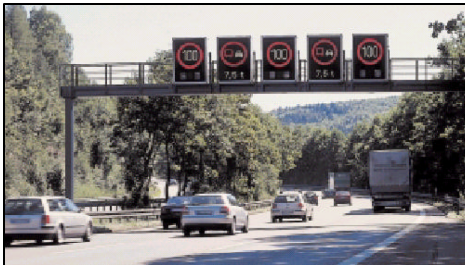
Figure 2-21. Overhead Gantry with Multiple VMSs on Autobahn 92 near Munich. 40
