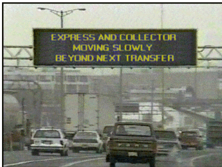
Figure 2-9. Large VMS Display in the Toronto Area. 28
