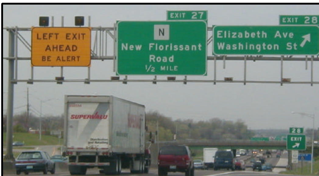
Figure 2-44. Left Exit Warning Sign in St. Louis, Missouri. 81
