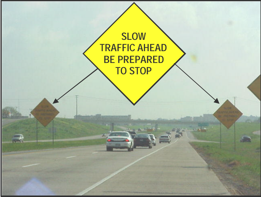
Figure 2-52. Southbound SH 121 Prior to Harwood Entrance – Slow Traffic Ahead Warning Signs.
