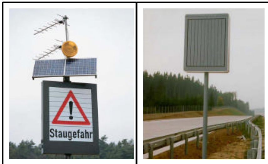
Figure 2-23. Variable Prism Panel Signs Used for Queue Warning in Germany. 38
