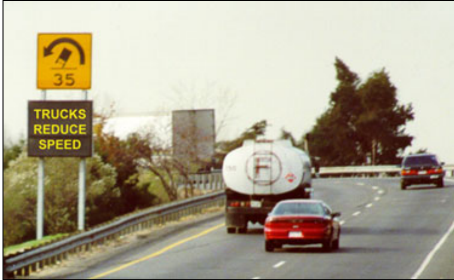
Figure 20. Active Warning System on the Capital Beltway.
