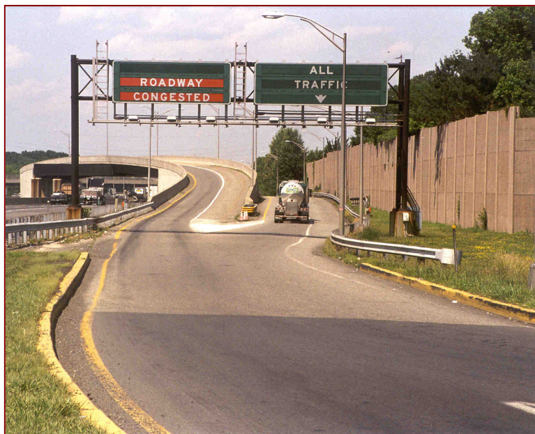
Figure 19. Variable Message Signs for Separate Roadways.
