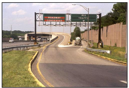
Figure 11. Individual Ramp Access for the Inner and Outer Roadways.
