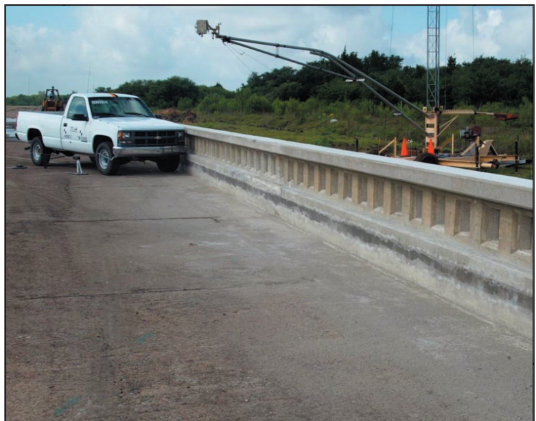
Texas F411 bridge rail with pickup truck
