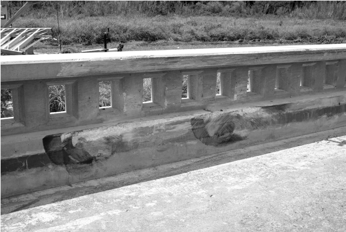
Figure 16. Installation after Test 442882-2.
