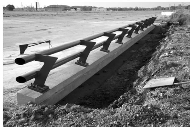
Figure 5. TxDOT F411 Bridge Rail before Test 442882-3 and 4.
