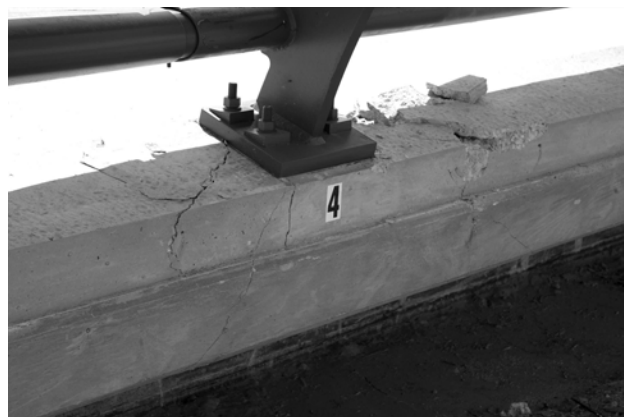
Figure 23. Installation after Test 442882-3.
