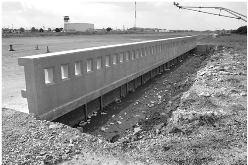
Figure 2. TxDOT F411 Bridge Rail before Test 442882-1.
