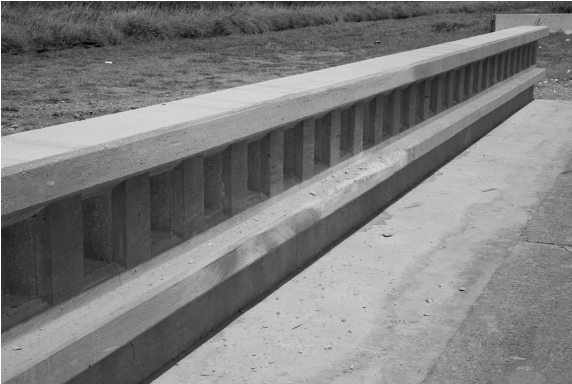
Figure 9. Installation after Test 442882-1.
