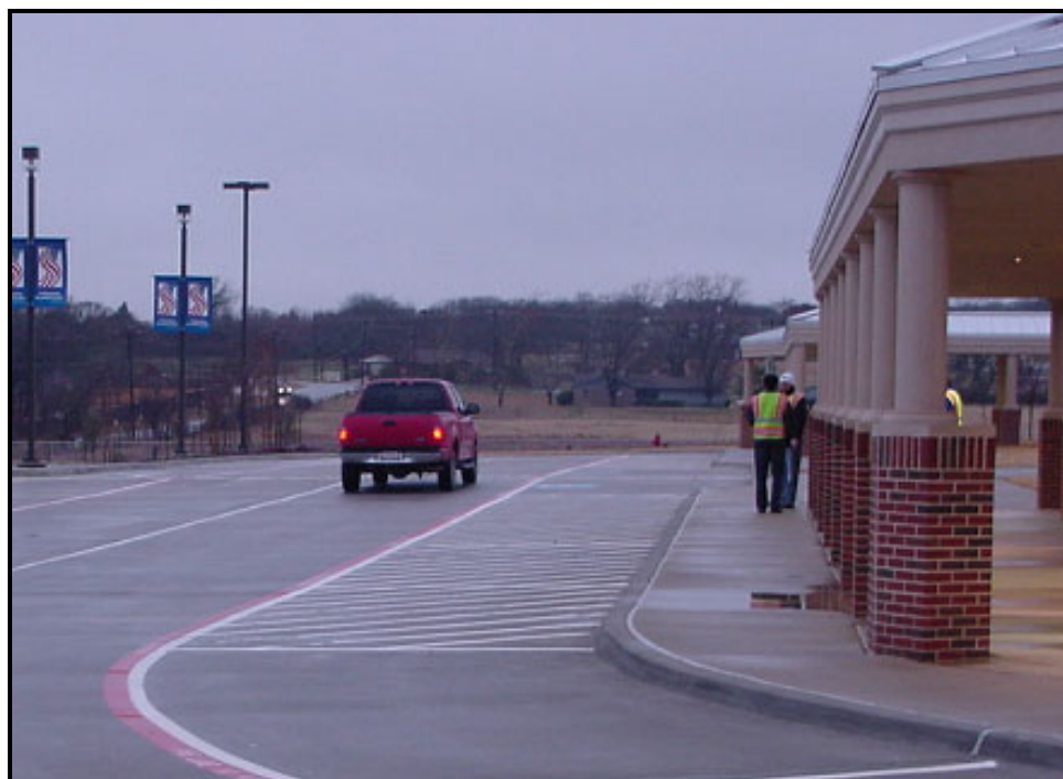
Figure 12. Covered Walkway Adjacent to the Parent Loading Zone.
