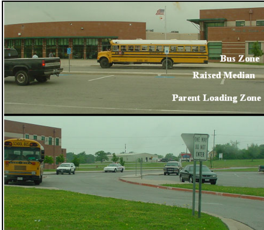
Figure 10. Site with a Layout to Avoid – Bus and Parent Zones Adjacent to Each Other.
