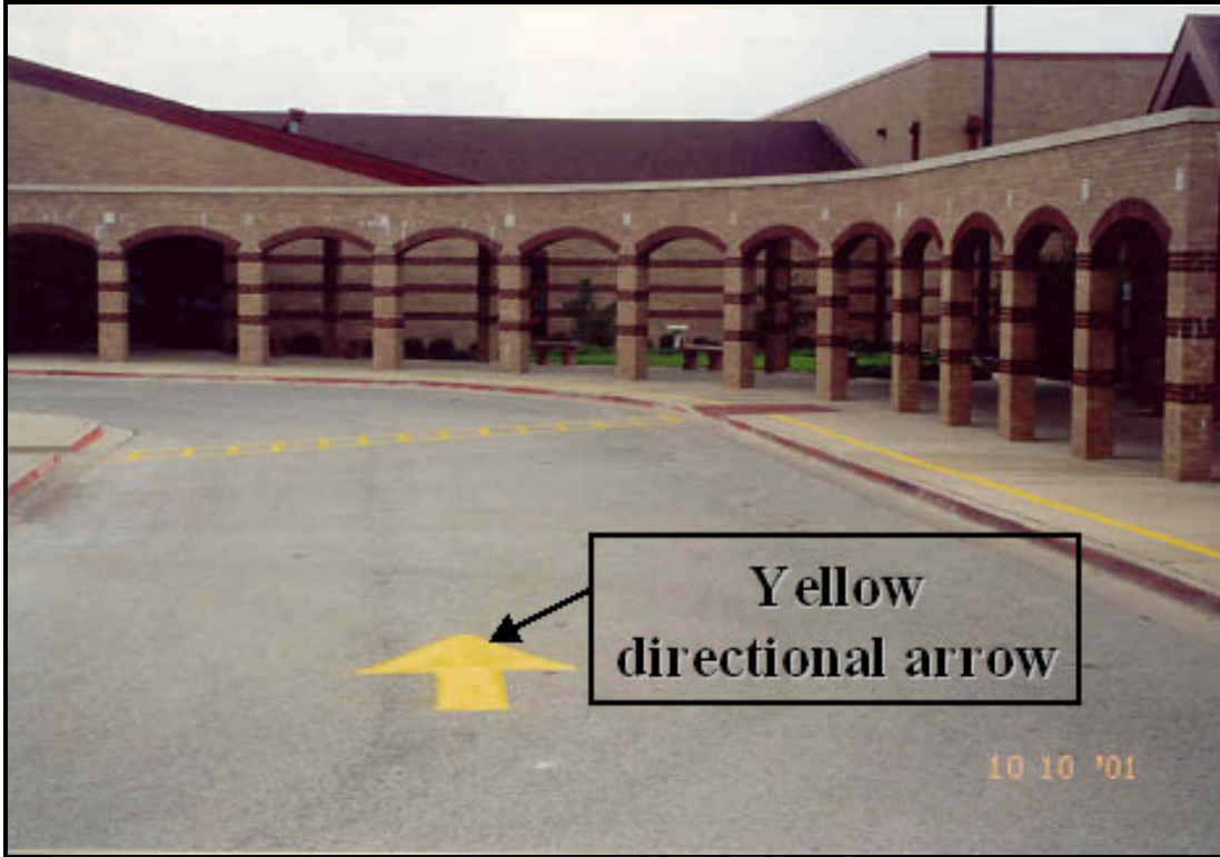
Figure 48. Example of Yellow Markings for On-Site Crosswalk at Elementary School.
