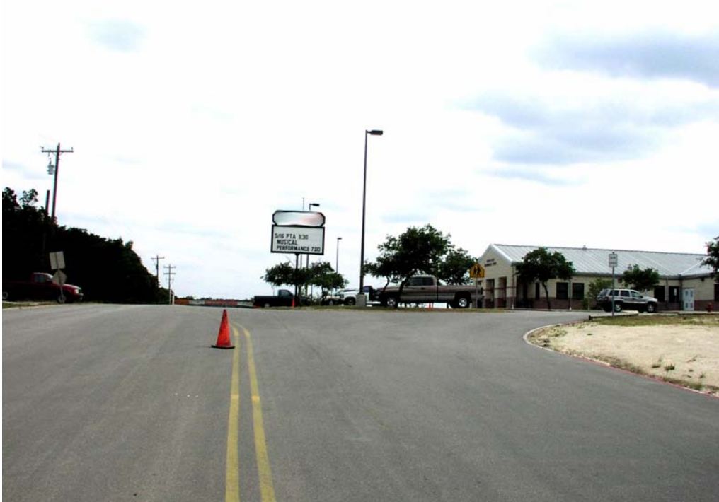
Figure 7-114. The Intermediate School Parent Drop-Off/Pick-Up Zone and Administration/Visitor Parking Lot (Facing South).
