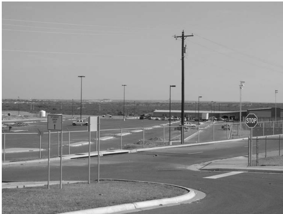
Figure 7-72. Employee Parking Lot Entrance/Exit (Facing Northwest).
