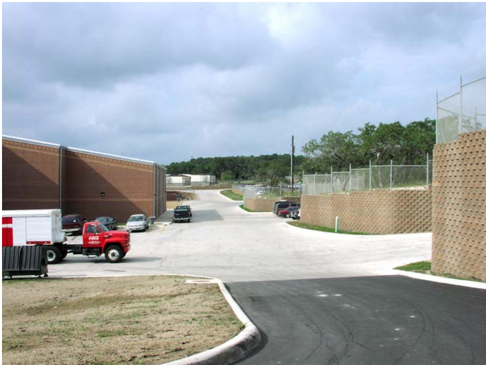
Figure 7-198. Service Roadway at the Rear of the School (Facing East).
