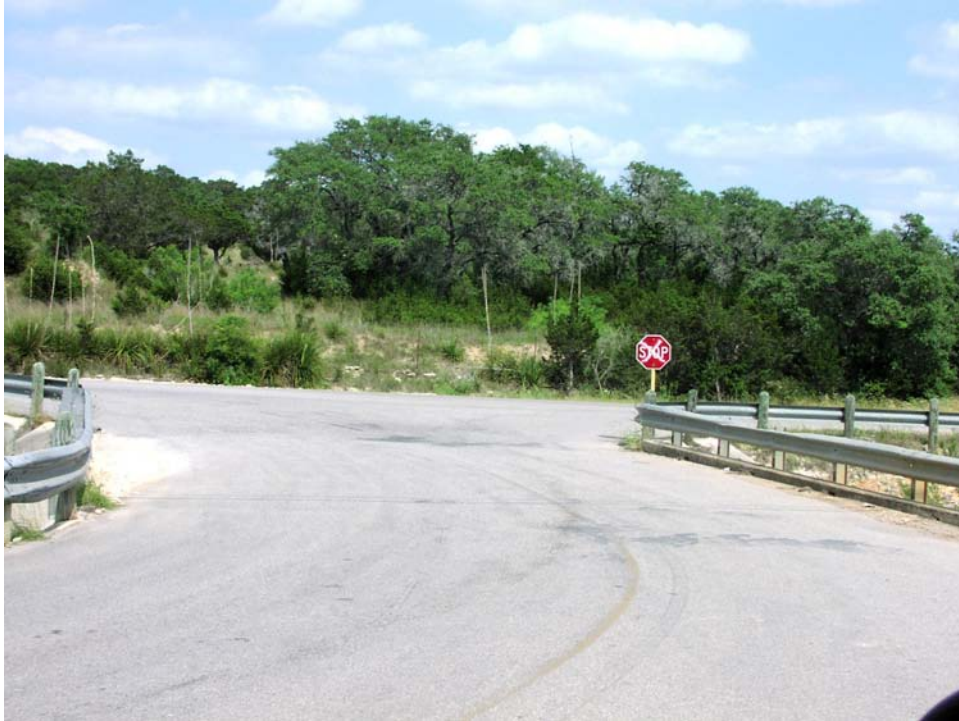
Figure 7-197. Driveway 3 (Facing East).
