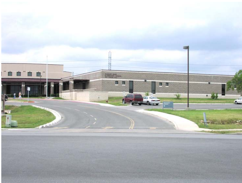
Figure 7-43. Driveway 1 (Facing North).
