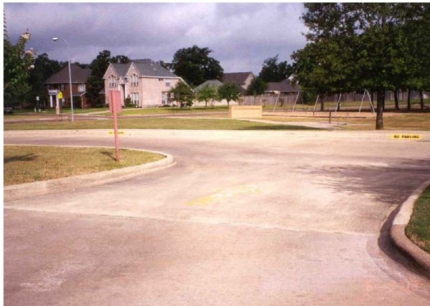
Figure 7-90. Exit Area of the Parking Area That Leads to the Exit Driveway in the Parent Drop-Off Zone.
