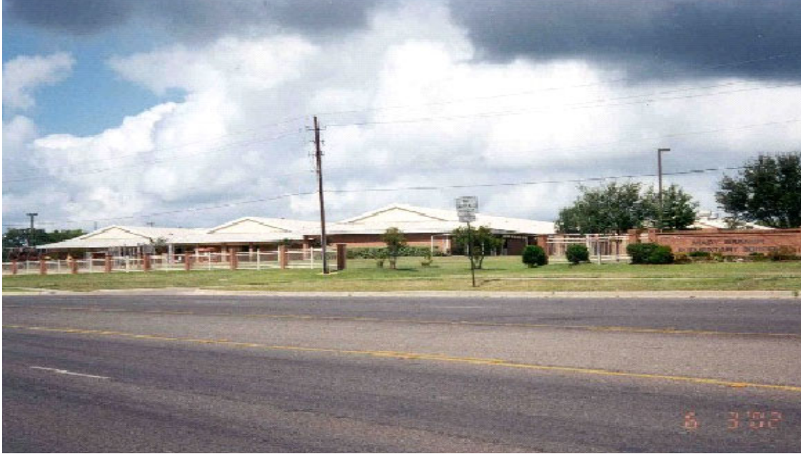
Figure 7-26. Front View of the Elementary School.
