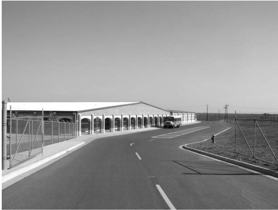
Figure 7-79. Driveway 4 and Eastside Drop-Off/Pick-Up Zone (Facing North).
