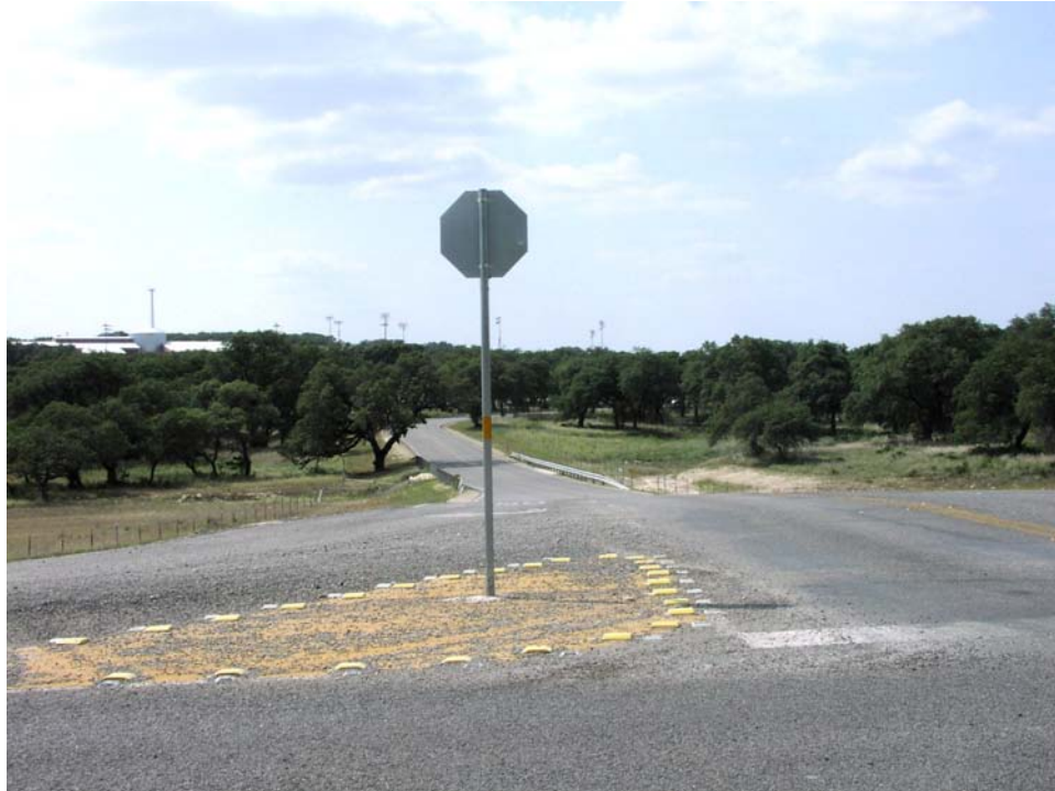
Figure 7-193. Driveway 2 (Facing West).
