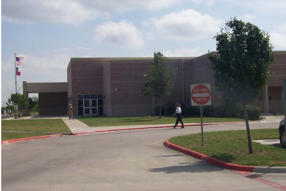
Figure 7-173. Drop-Off Zone in the Faculty Parking Lot at the Middle School.
