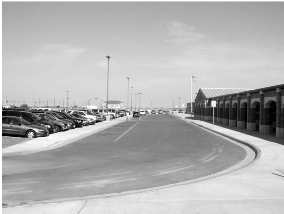
Figure 7-76. Drop-Off/Pick-Up Zone in Front of School (Facing West).
