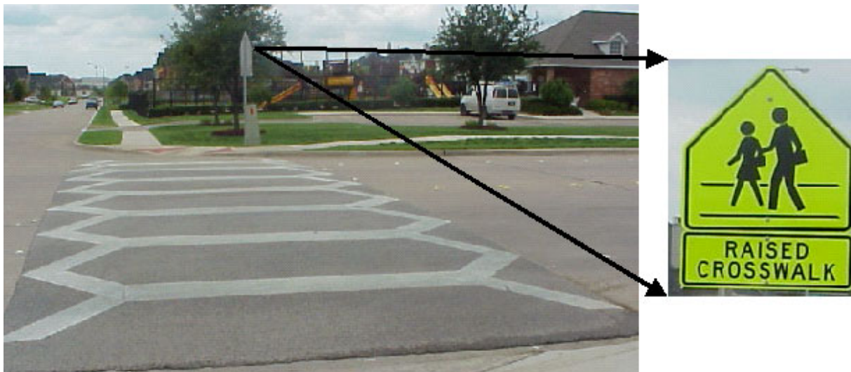
Figure 7-21. Raised Crosswalk across the Minor Collector Roadway in Front of the School.
