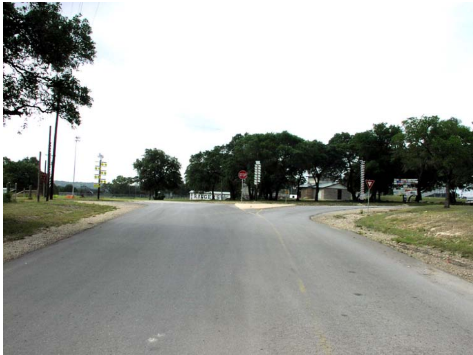
Figure 7-192. Driveway 1 at Three-Leg Intersection (Facing South).
