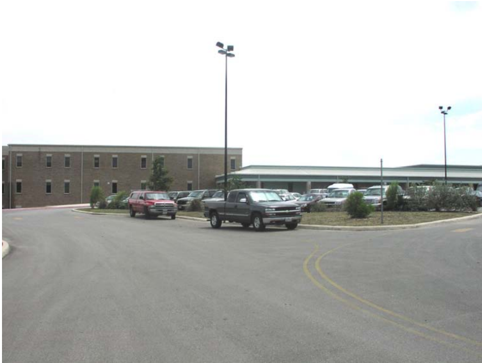
Figure 7-132. Administration/Visitor Parking Lot (Facing South).
