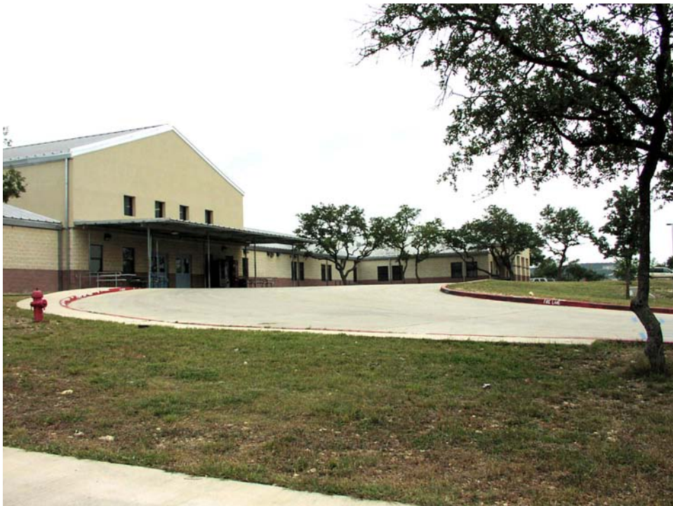
Figure 7-117. The Intermediate School Bus Drop-Off/Pick-Up Zone (Facing Northwest).
