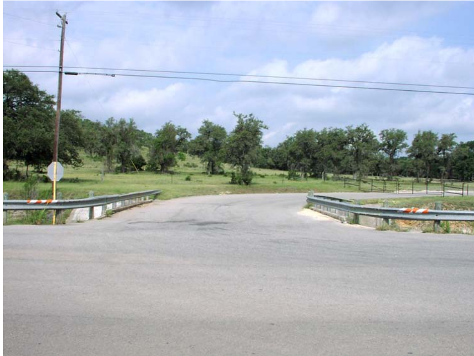
Figure 7-196. Driveway 3 (Facing West).
