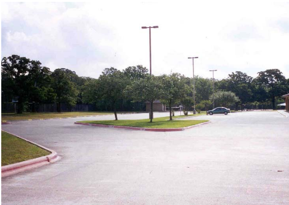
Figure 7-97. The Faculty/Bus Parking Lot.
