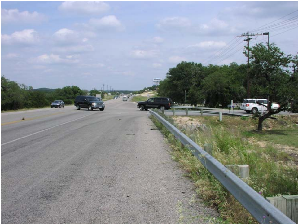
Figure 7-103. Driveway 1 (Facing East).
