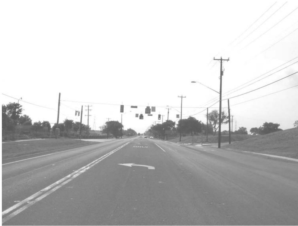
Figure 7-219. The FM Road and Driveway 3 Intersection (Facing Southeast).
