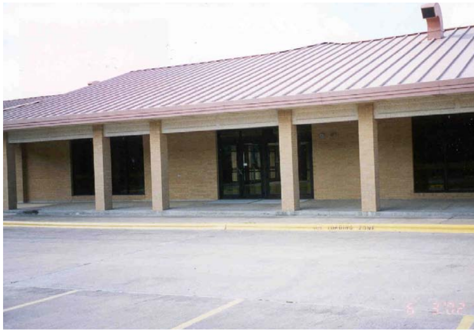
Figure 7-96. Bus-Loading Zone in Bus/Faculty Parking Lot.
