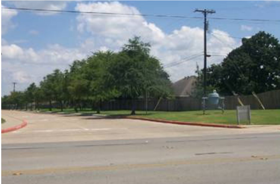
Figure 7-161. Entrance and Exit Driveway to the Drop-Off Parking Lot.
