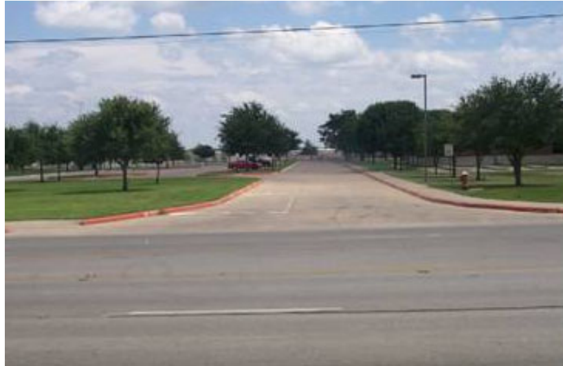
Figure 7-152. Entrance and Exit Driveway to the Bus/Faculty Parking Lot.
