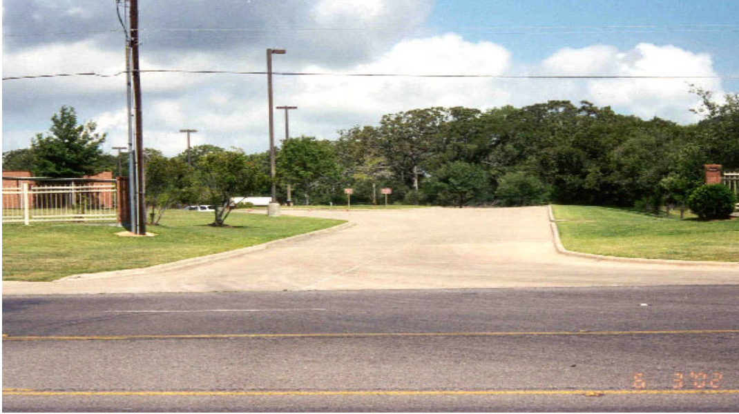
Figure 7-36. Entrance and Exit Driveway to the Bus Parking Lot.
