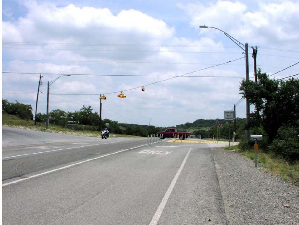
Figure 7-205. Student Disregarding the No Left Turn Restriction at Driveway 1.
