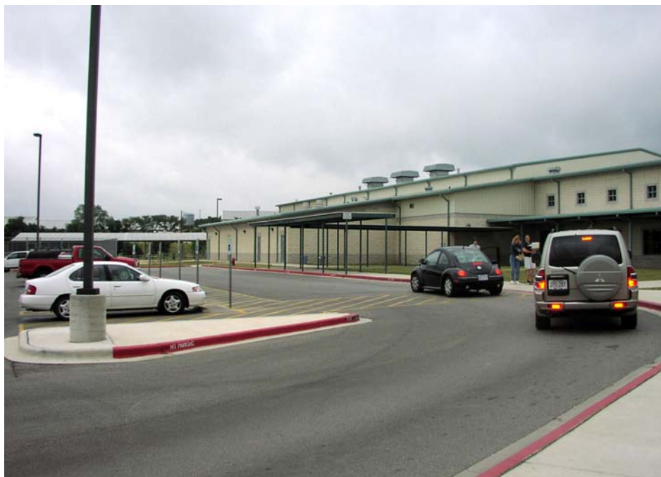
Figure 7-109. The Middle School Parent Drop-Off/Pick-Up Zone (Facing South).
