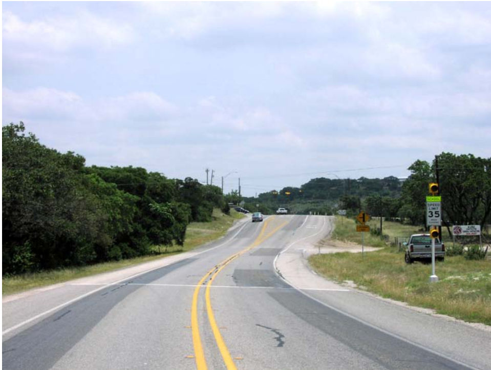
Figure 7-187. Eastbound Approach to the High School (Facing East).
