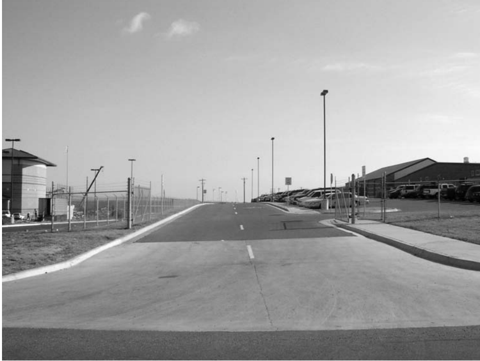
Figure 7-69. Driveway 1 (Facing North).
