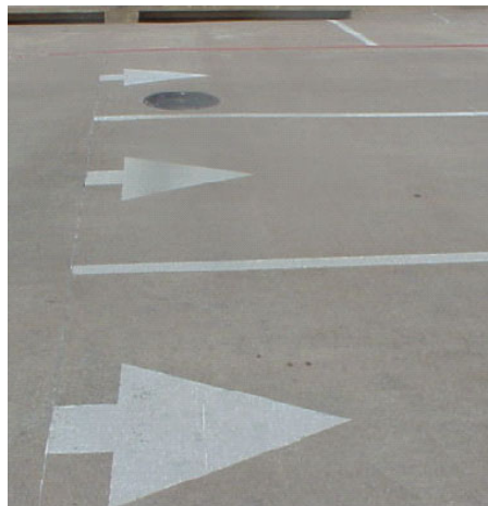
Figure 7-19. Pavement Markings at the Start of the Parent Drop-Off/Pick-Up Zone.
