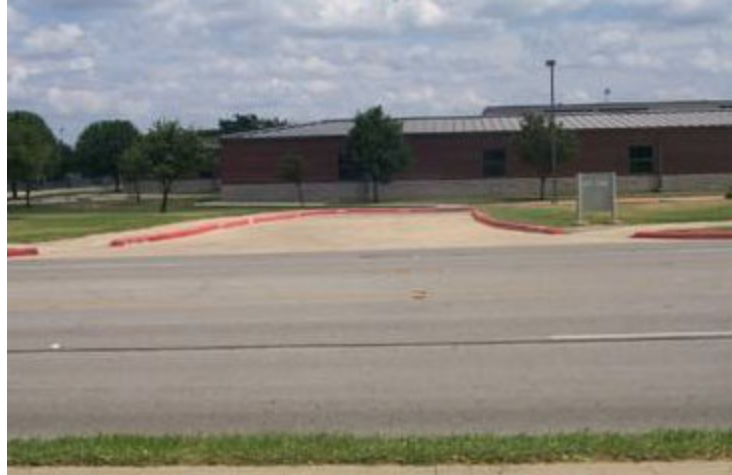
Figure 7-159. The Exit to the Visitor Semicircle, Driveway 2.
