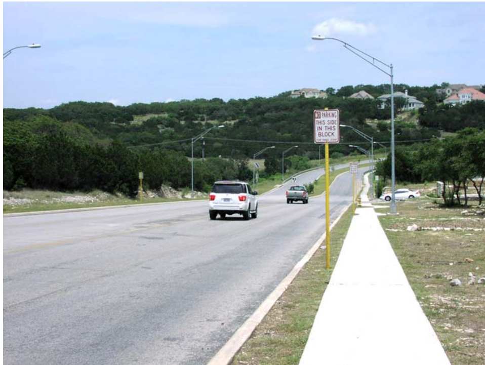
Figure 7-127. Parking Restriction Signing (Facing Northeast).
