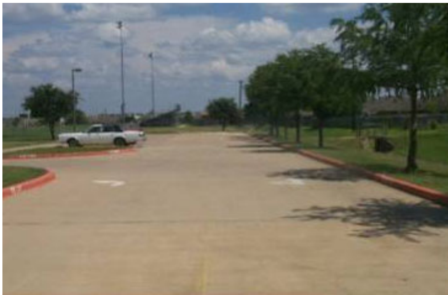
Figure 7-162. Arrows Illustrating the Options of Continuing to the Drop-Off Loop or Parking Area.
