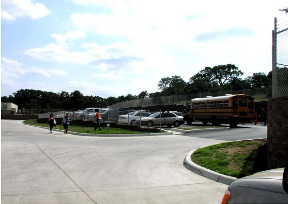
Figure 7-199. Bus Drop-Off/Pick-Up Zone (Facing East).
