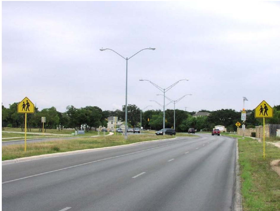
Figure 7-42. Road Signing (Facing Northeast.)
