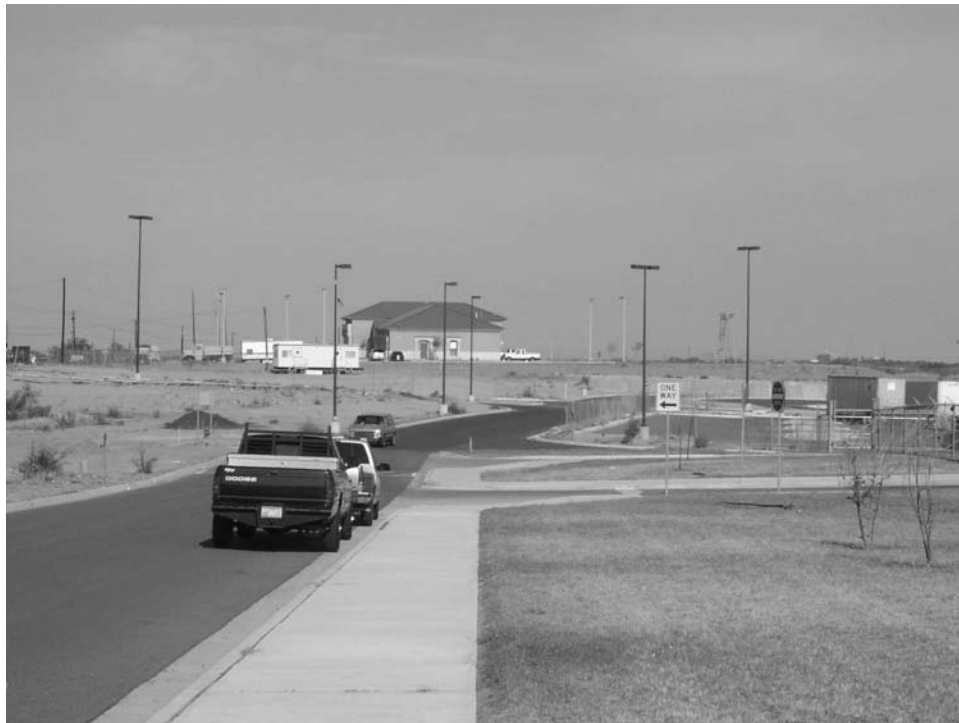
Figure 7-78. Driveway 3 (Facing West).
