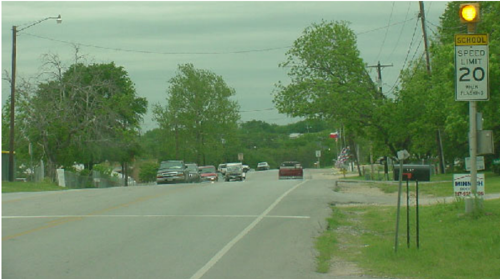
Figure 7-6. School Zone on Northbound Approach.
