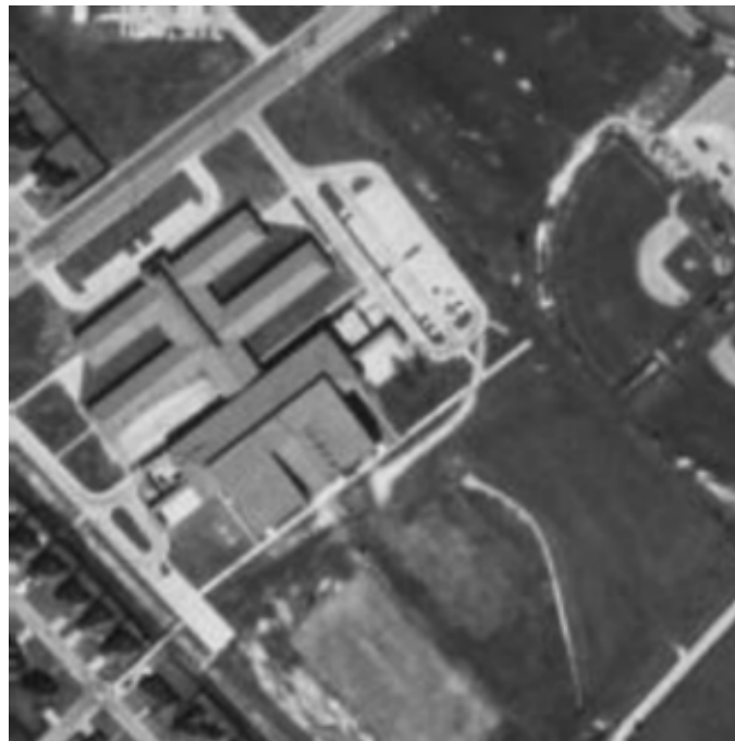
Figure 7-150. Aerial View of the Middle School Case Study Site 3 (47).
