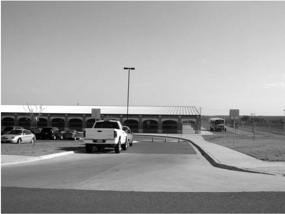
Figure 7-73. Driveway 2 (Facing North).
