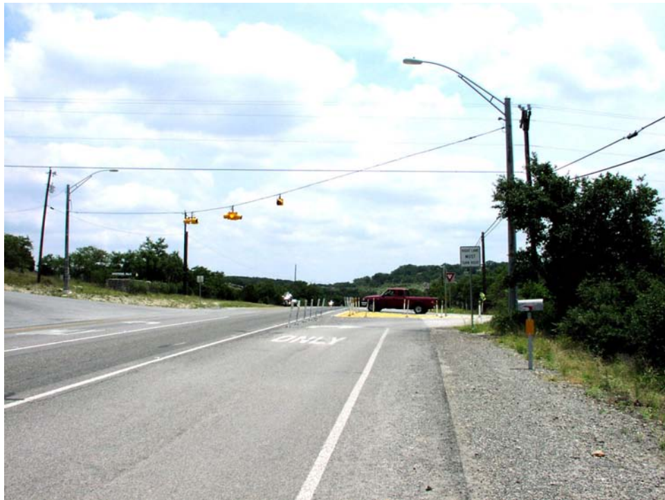
Figure 7-190. Driveway 1 (Facing East).
