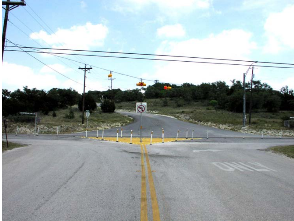
Figure 7-191. Driveway 1 (Facing North).
