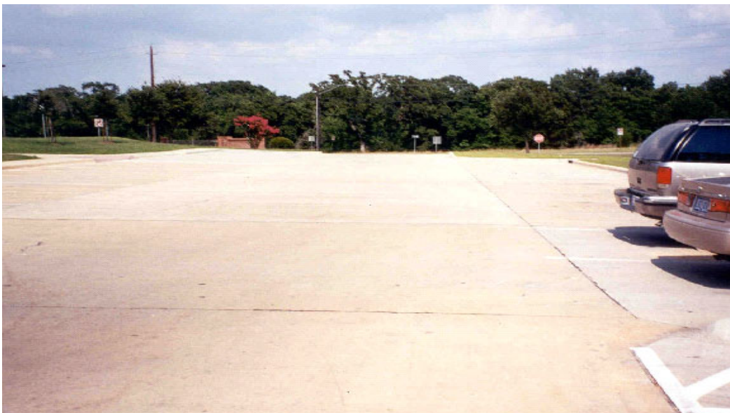
Figure 7-31. The Farthest Parking Area to the School in the Parent Drop-Off Parking Zone.
