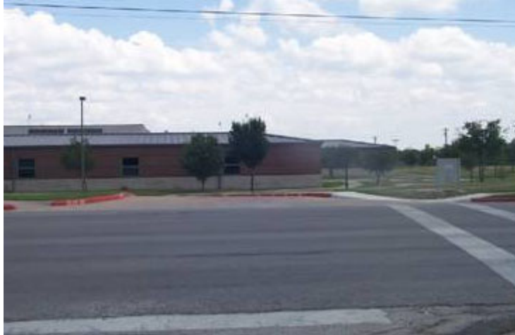
Figure 7-157. Entrance Driveway to the Visitor Semicircle.
