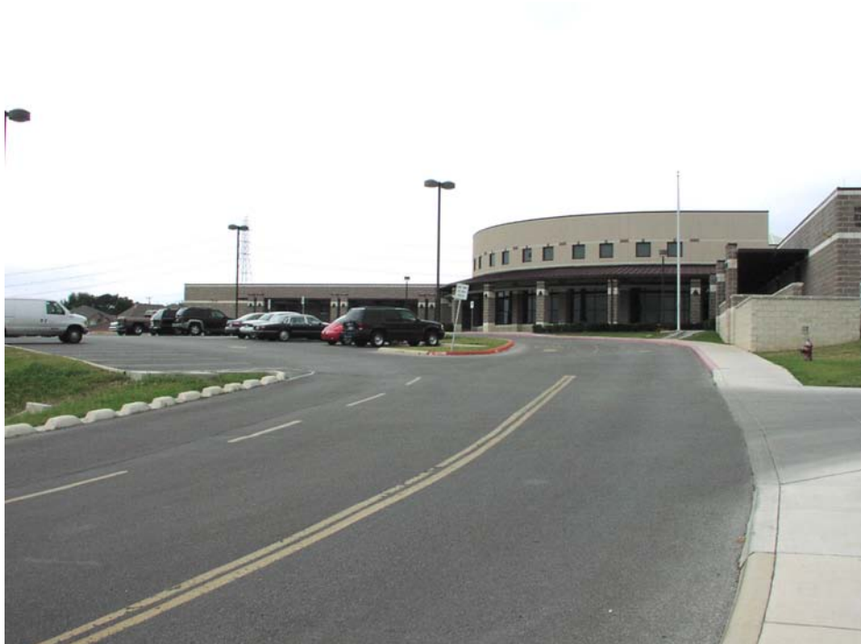
Figure 7-46. The Entrance to the Parent Drop-Off/Pick-Up Zone, and Exit from the Drop-Off Zone and West Administration/Visitor Parking Lot (Facing Northwest).
