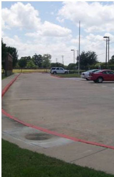
Figure 7-158. A View of the Through Lane and Parking Area in the Visitor Semicircle.
