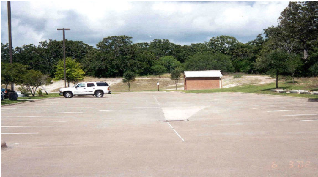
Figure 7-37. Parking Area in the Bus Parking Lot.
