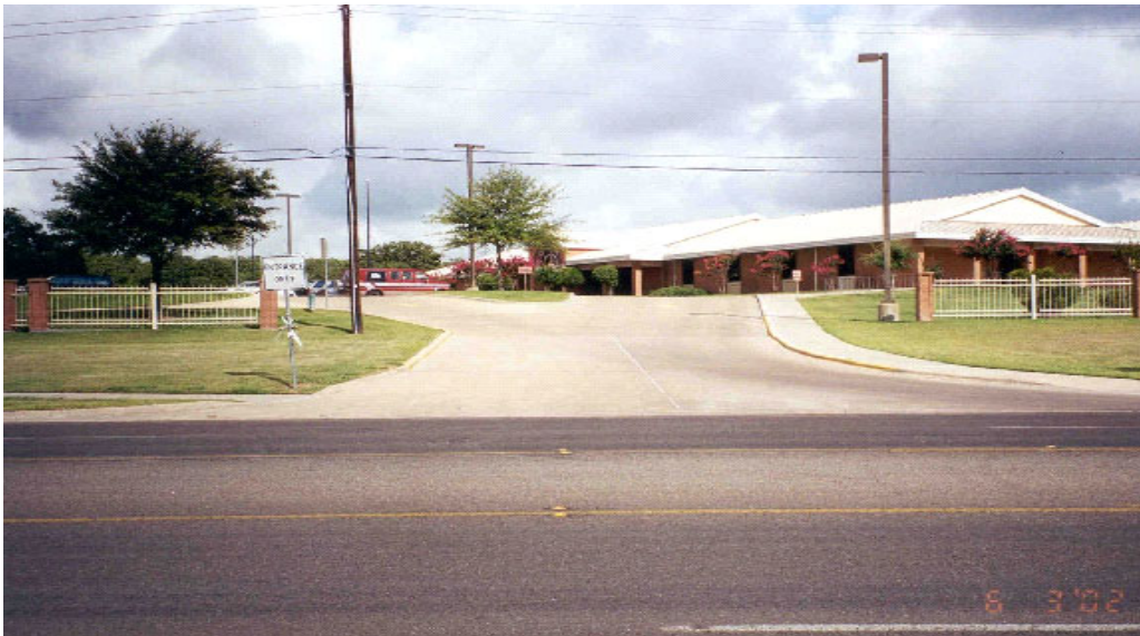
Figure 7-27. Entrance Driveway to the Parent Drop-Off Zone.
