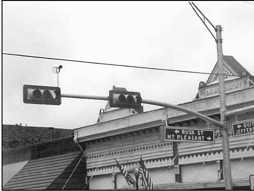
Figure 2-8. Mast Arm Camera Mount.
