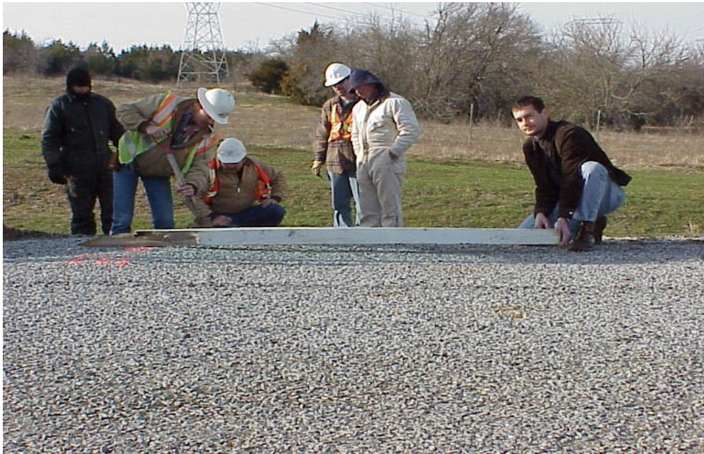
b. U.S. 82 Newly Constructed Section, West of Sherman (2002).
