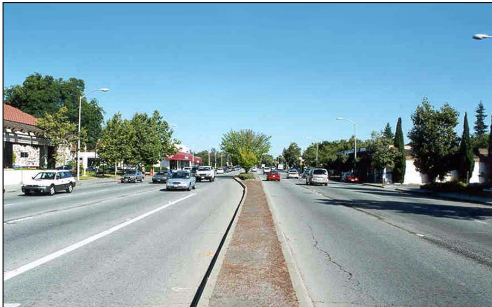
Figure 25. State Route 82 in Palo Alto before improvements.
