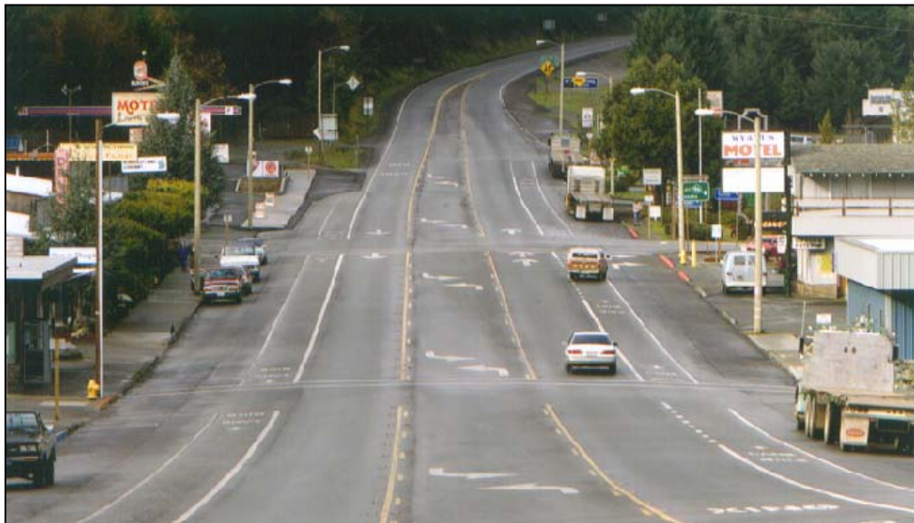
Figure 31. State Route 299, Willow Creek, after re-striping.
