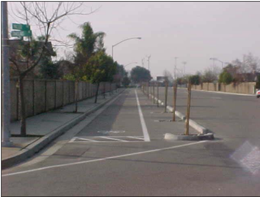
Figure 29. Escalon after roadway improvements.
