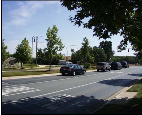
Figure 23. Kentlands Blvd at MD 119 is a major, signal-controlled intersection.
