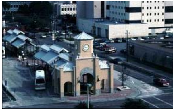
Figure 6. The Staples Street Bus Station in Corpus Christi, a low-cost transportation project, improved access and helped revitalize the surrounding area. Source: Project for Public Spaces ( www.pps.org )
