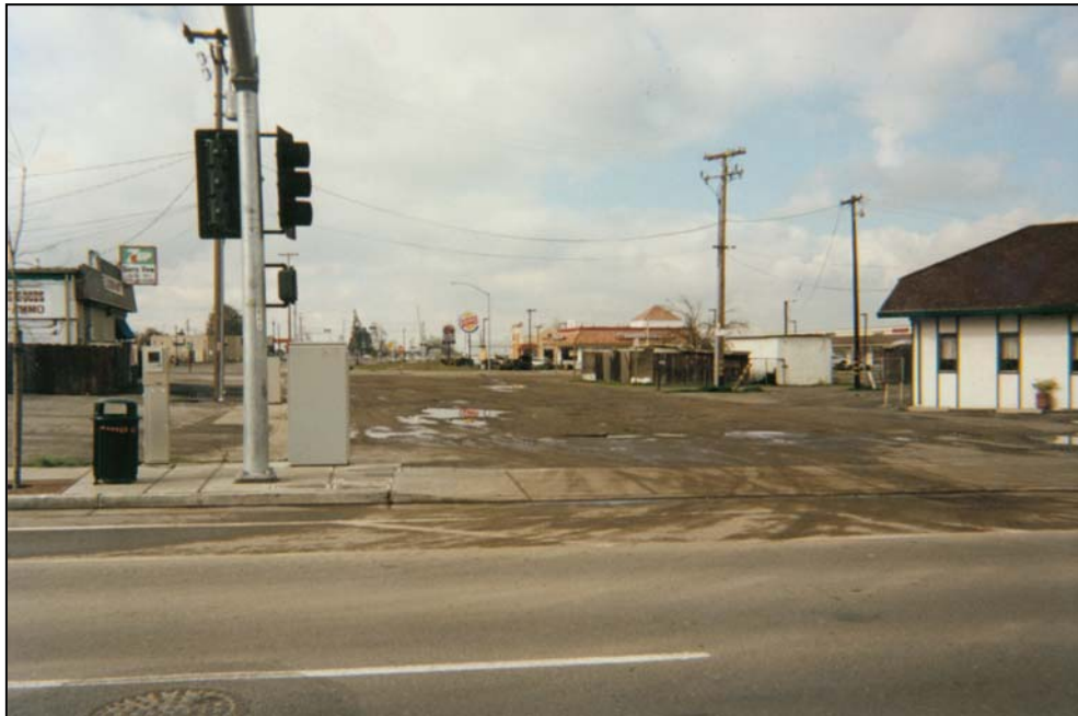
Figure 28. Escalon before roadway improvements.
