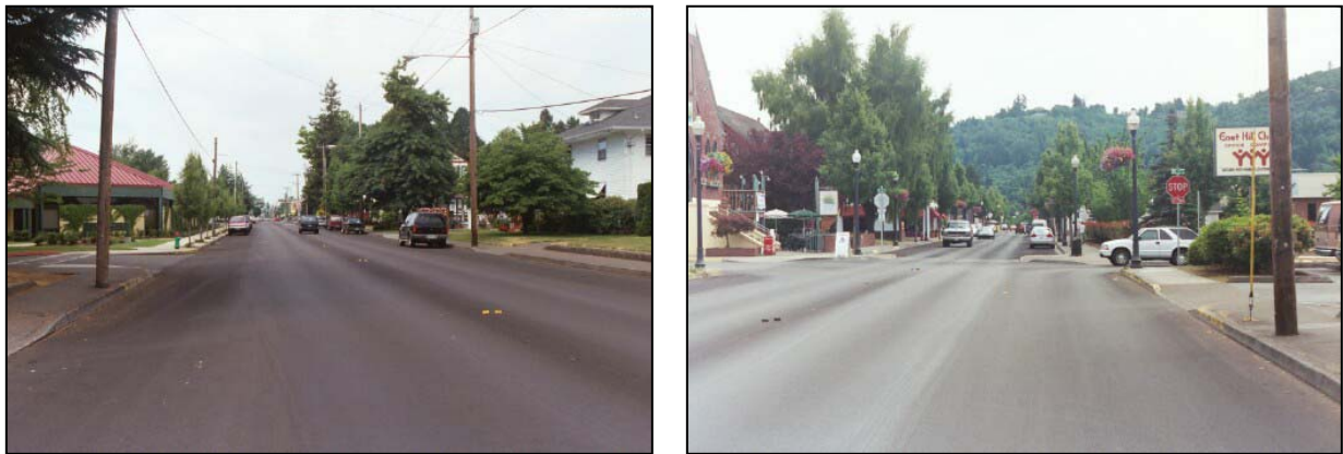
Figure 47. Main Street was converted from four lanes with parking (left photo) to two lanes with parking and wider sidewalks (right background photo) in Gresham.
