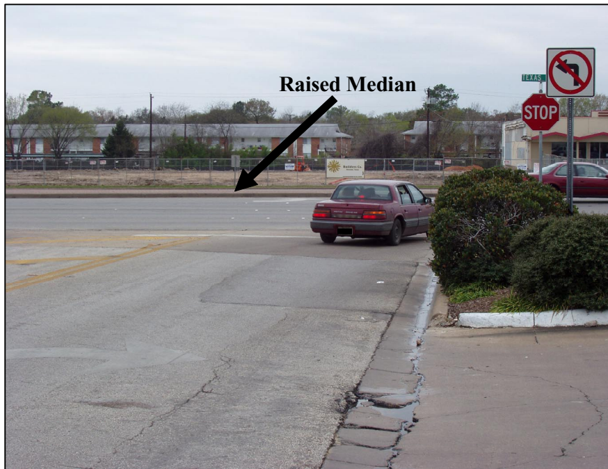
Figure 3-10. Raised Median Restricting Left Turns at Dominik Drive.
