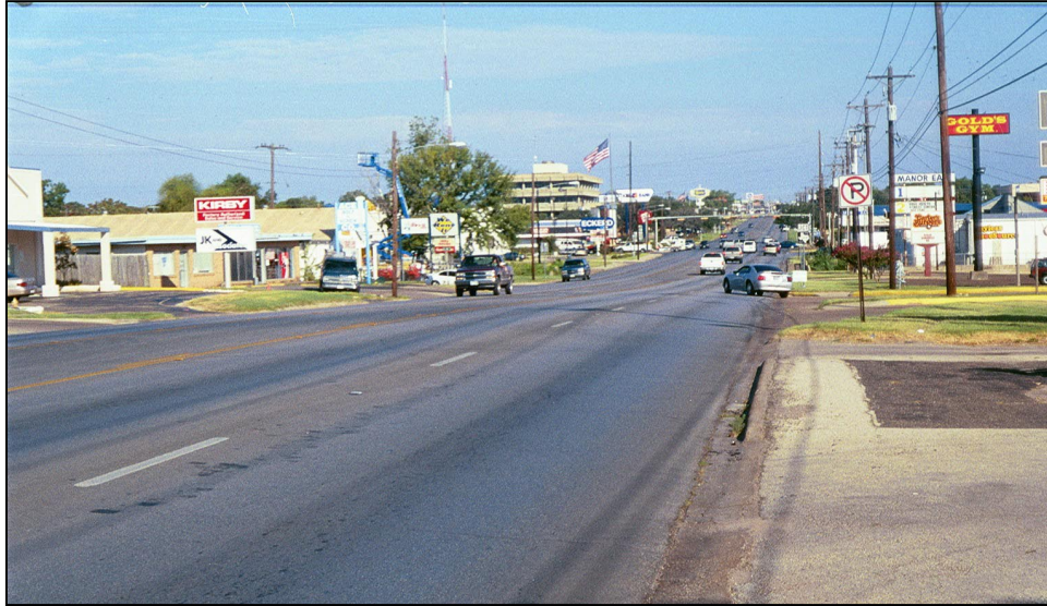
Figure 2-3. Texas Avenue Facing North with Villa Maria in the Background.
