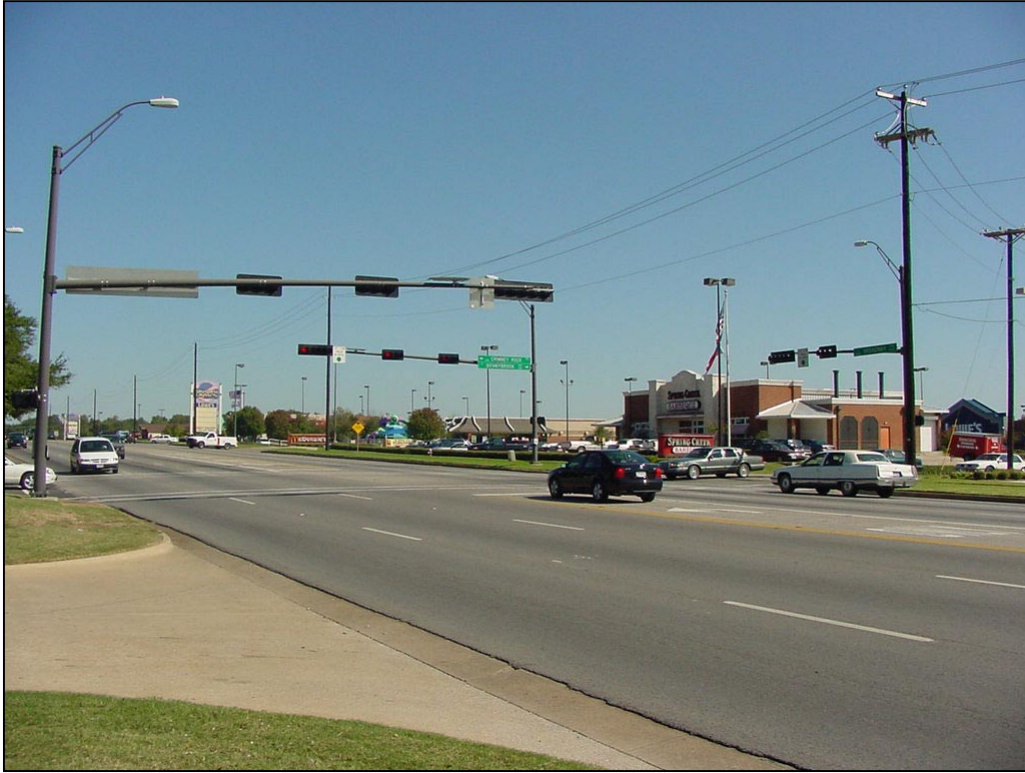
Figure 2-7. Broadway Avenue Facing North to Chimney Rock Signalized Intersection.
