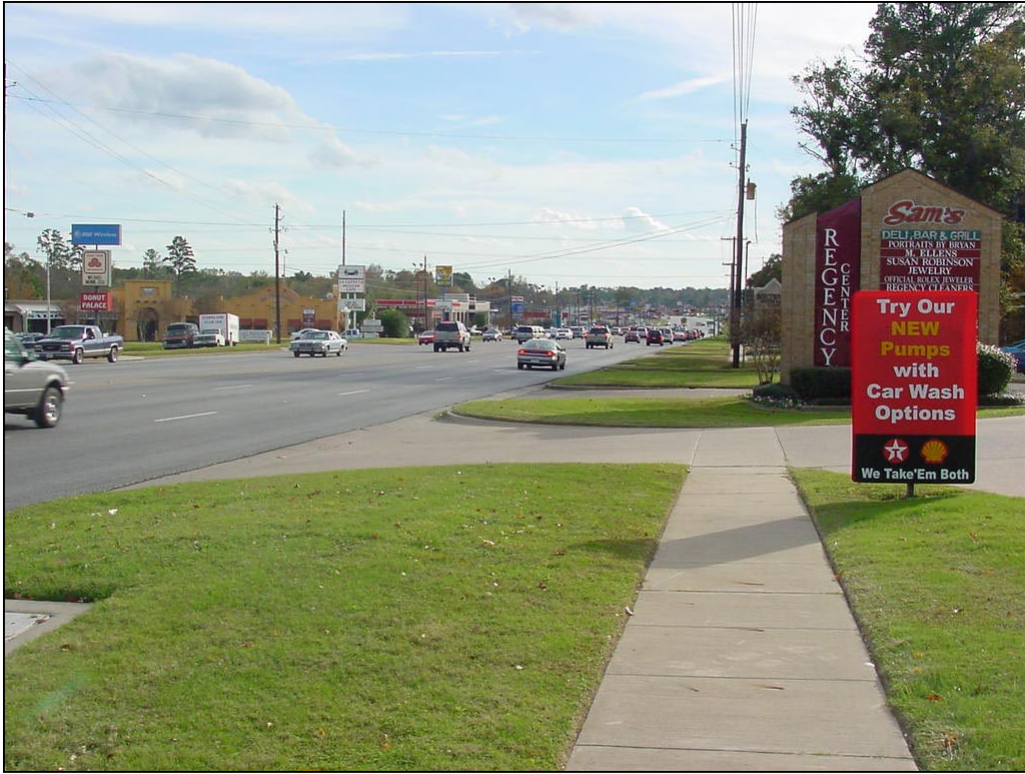
Figure 2-8. Broadway Avenue Facing South at Chimney Rock Signalized Intersection.
