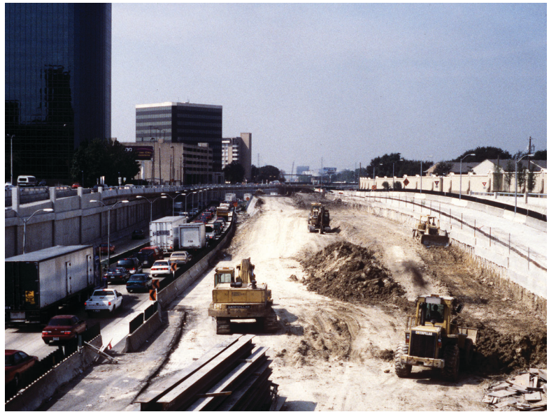
Figure 1. A major freeway reconstruction in an urban area
