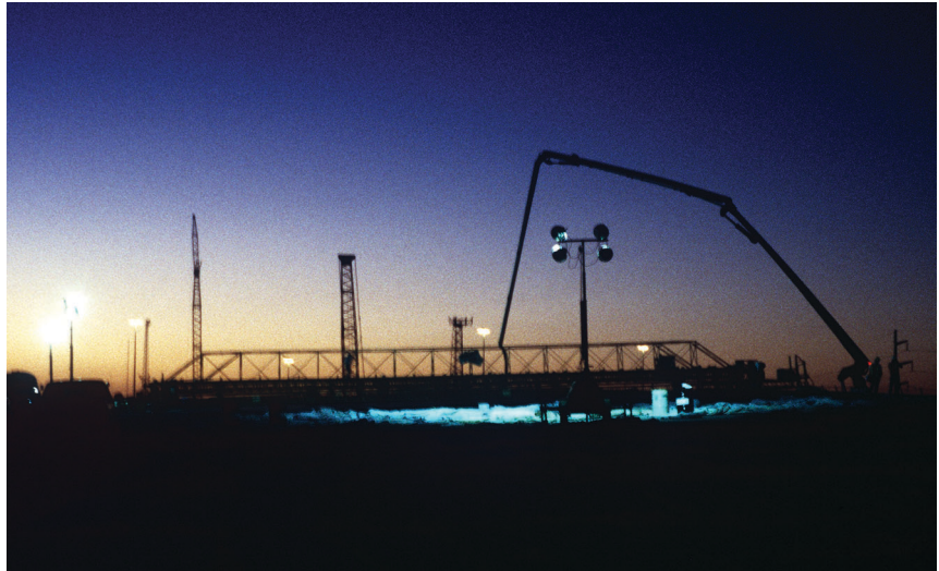
Figure 2. Early morning elevated concrete placement
