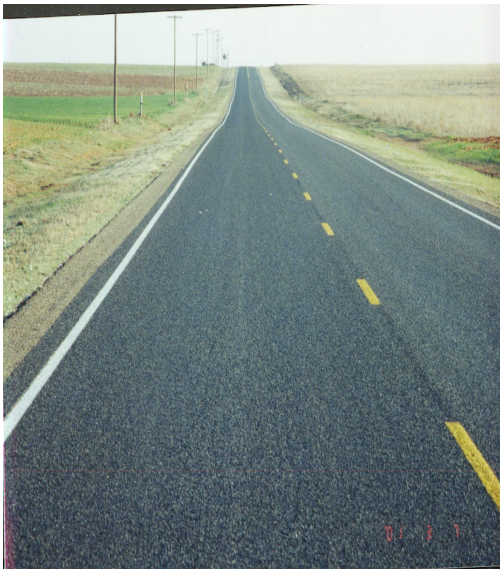
Figure 22. FM 301 10% Fly Ash Excellent Condition.
