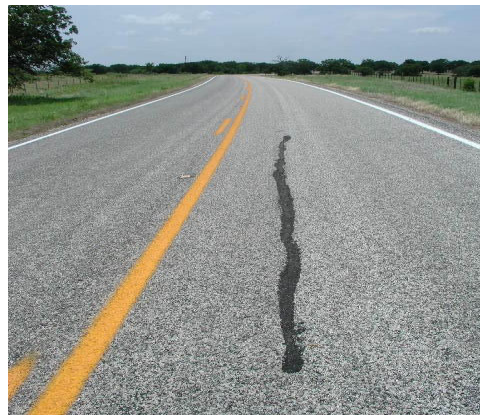
Figure 16. Longitudinal Cracking in Control Section (no grid) of FM 1915 after 3 Years in Service.
