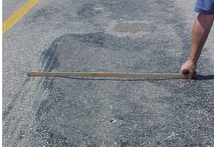
a) Section 1 Roadbond Treated
