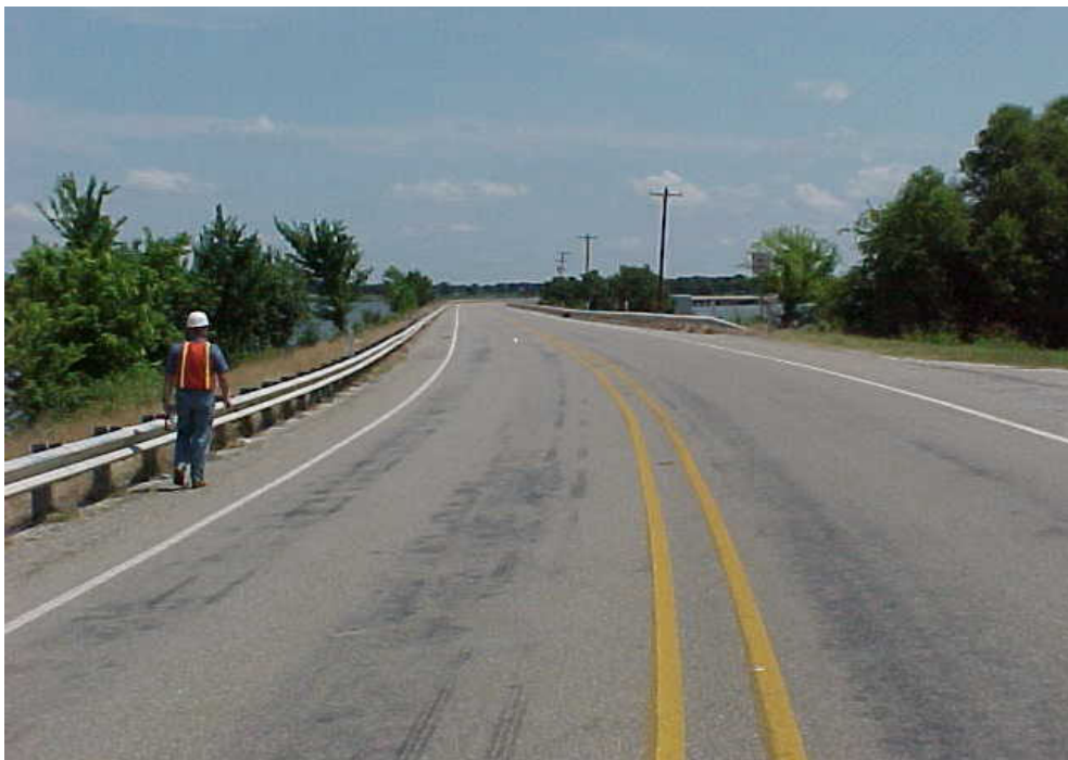
Figure 39. View of Sections 1, 2, and 3 in June 2002.
