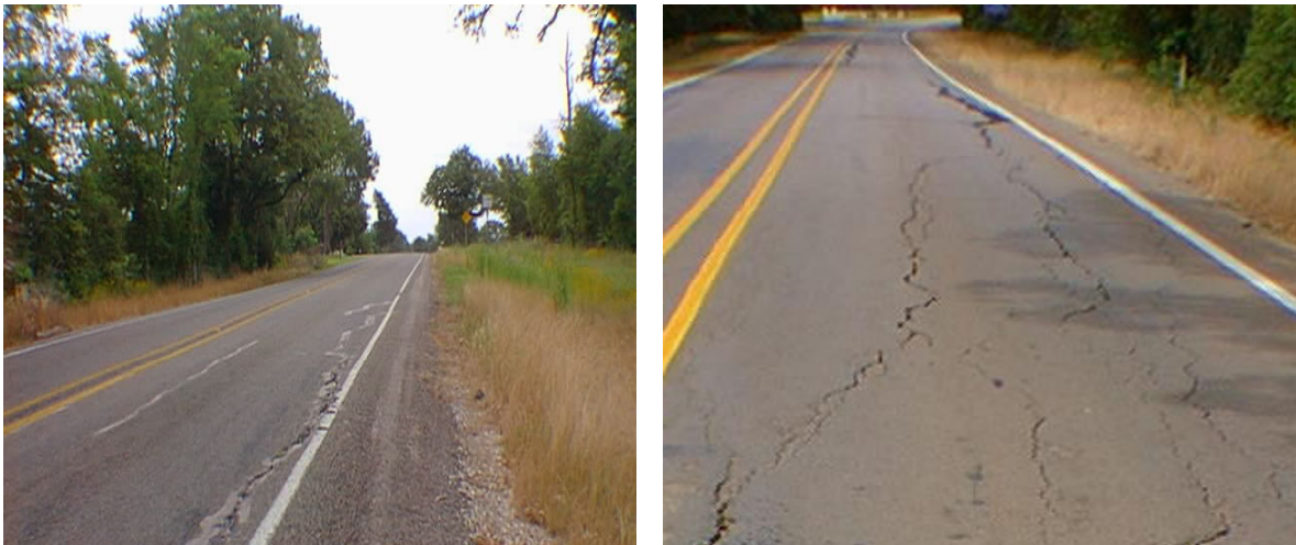
Figure 13. Severe Longitudinal Cracking Problems in Some of the Initial Recycled Pavements in the Bryan District.
