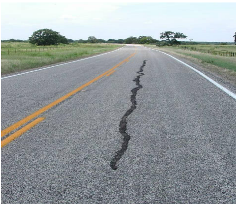
Figure 16. Longitudinal Cracking in Control Section (no grid) of FM 1915 after 3 Years in Service.
