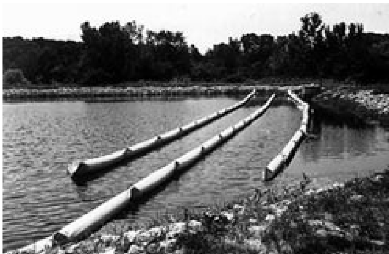
Figure 4. Containment Boom, Advanced Environmental Systems, Inc.
