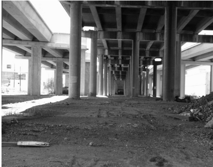
Figure 18. SH 59 at IH-10 Downtown Stockpile and Dump Area Close to Enron Field. Approximately 0.2 of a mile of available space beneath elevated section of SH 59.
