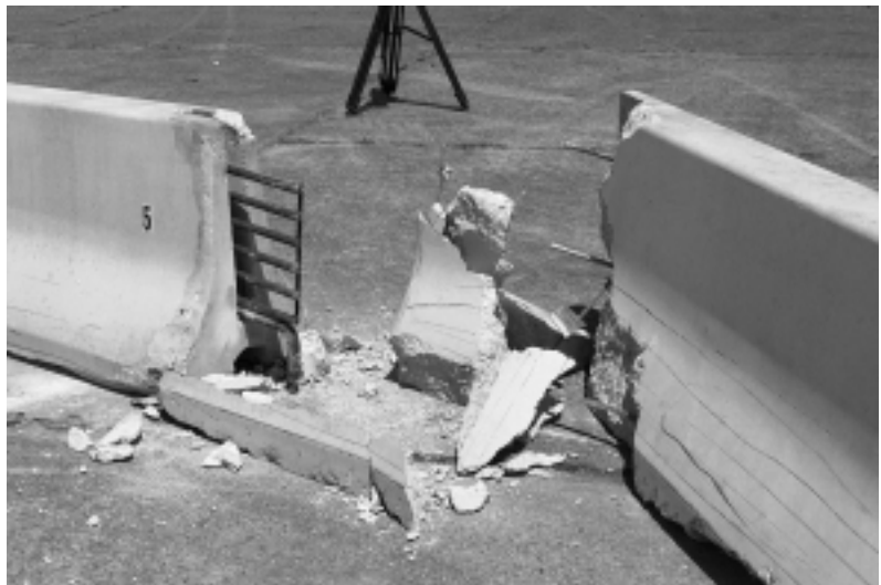
Figure 16. Installation after Test 441621-2.
