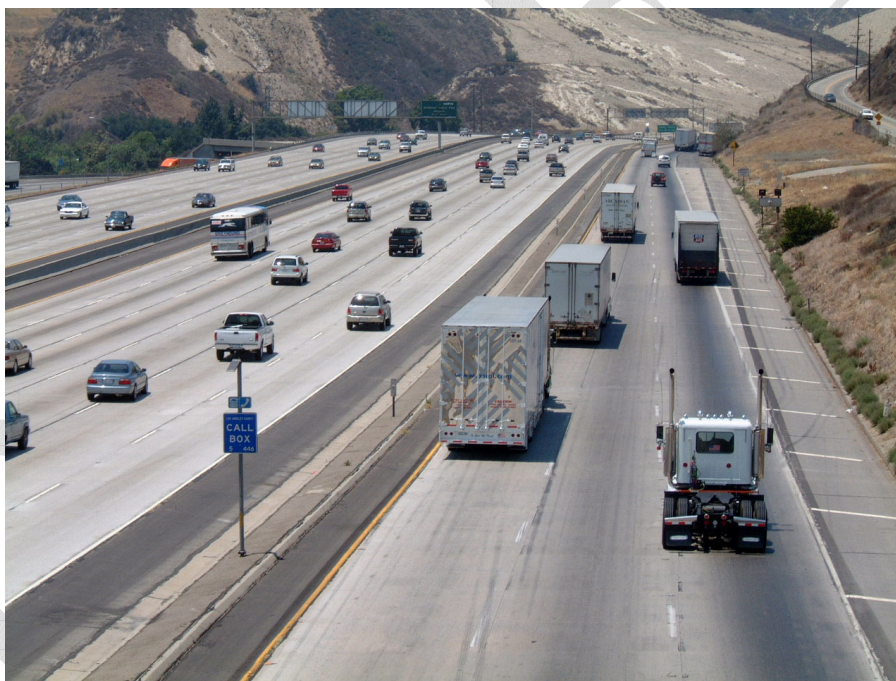
Figure 2-8. IH-5 Truck Roadway, Los Angeles, California.
