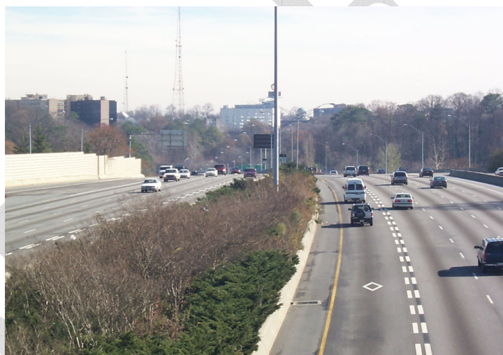
Figure 2-5. IH-75 Contraflow HOV Lane, Atlanta, Georgia (5).
