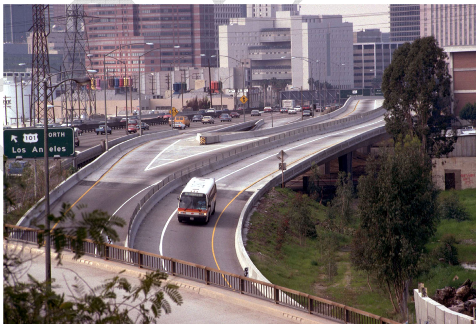
Figure 2-1. IH-10 (El Monte) Two-Way, Barrier-Separated HOV Lane, Los Angeles, California (5).
