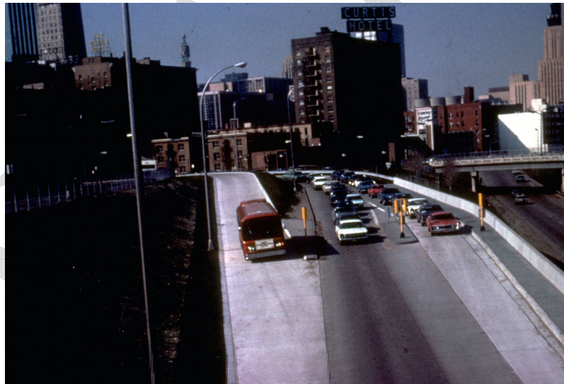
Figure 2-9. Ramp Meter Bypass Lane, Minneapolis, Minnesota (5).
