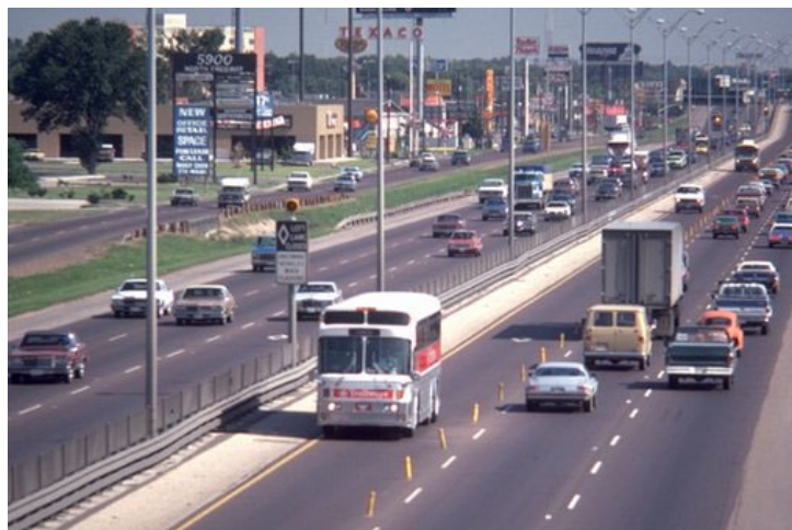
Figure 2-4. IH-45 (North) Contraflow HOV Lane, Houston, Texas (5).
