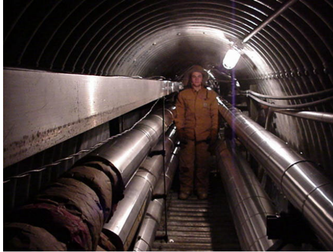
Figure 2-6. Utilidor Walkway (20).
