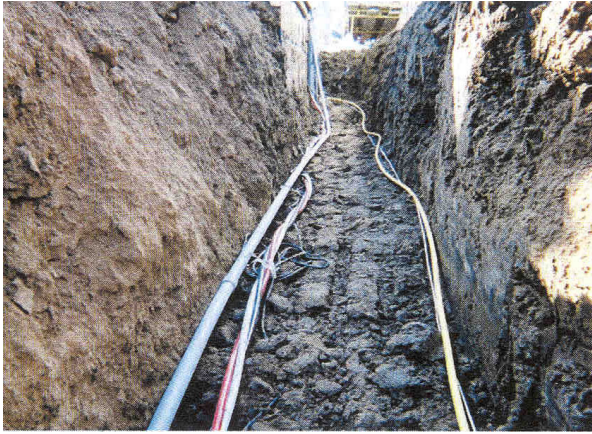
Figure 6-1. Joint Trench Installation.
