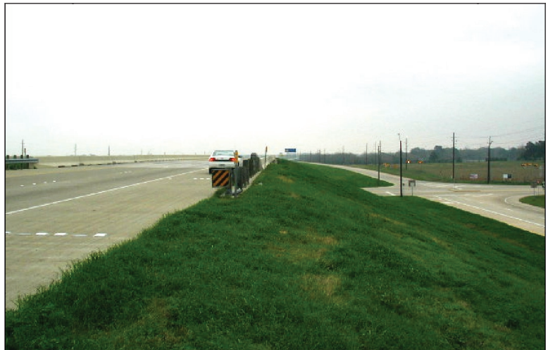
Figure 1. An Example of Bridge Approach Slab (US 290 at FM 362).
