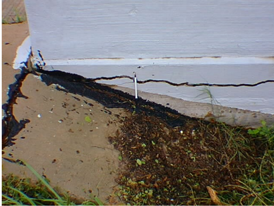
Figure 4.2. Side View of SH99 at Oyster Ck.
