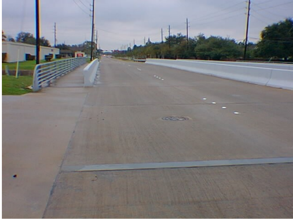
Figure 4.4. FM1876 at A22 Ditch.
