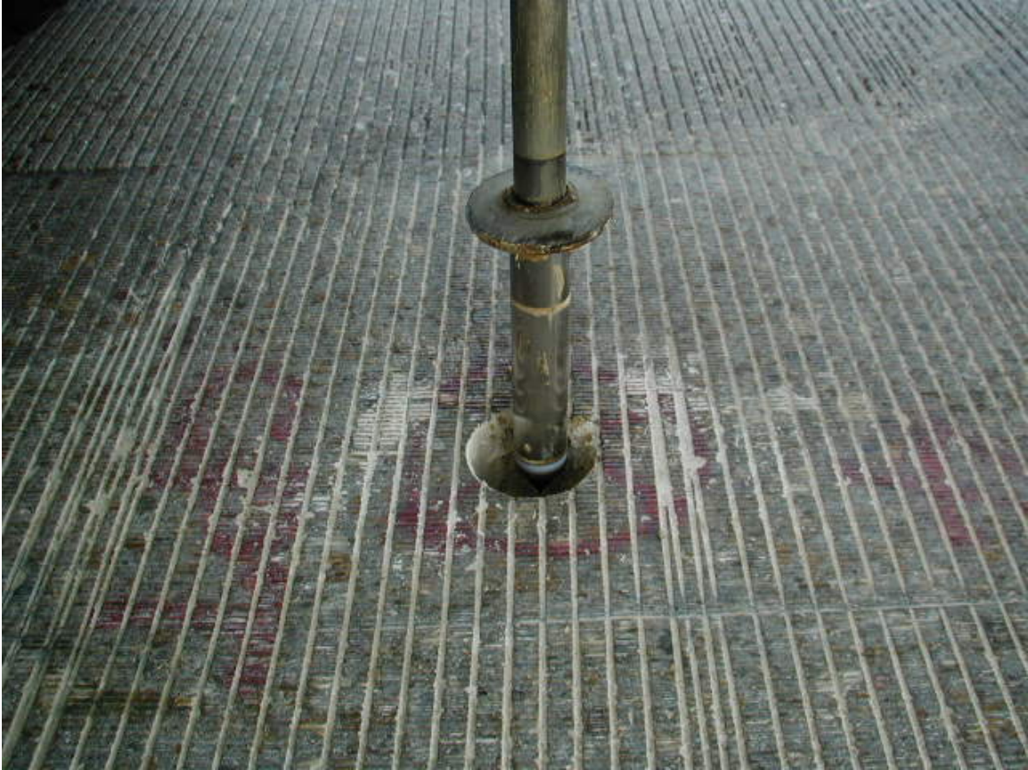
Figure 7.9. CPT Cone Right before Penetration.
