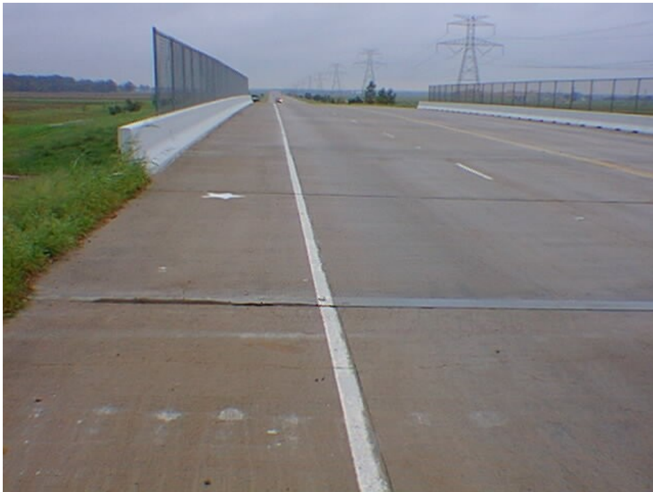
Figure 4.1. Front View of SH99 at Oyster Ck.
