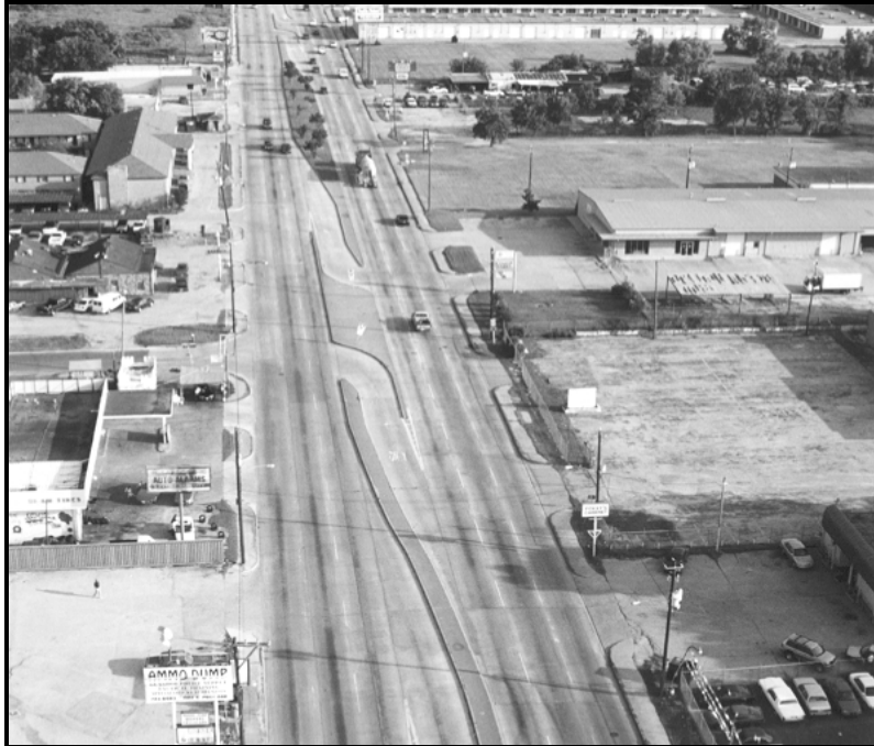
Figure 3-15. Directional Median Opening in Houston, Texas.
