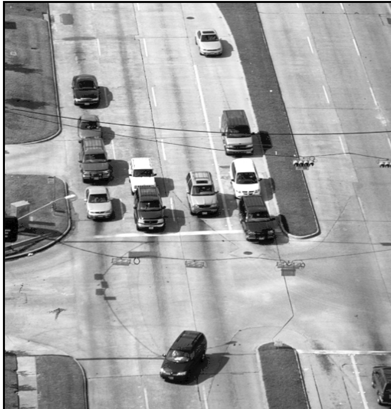
Figure 3-13. Insufficient Corner Clearance.
