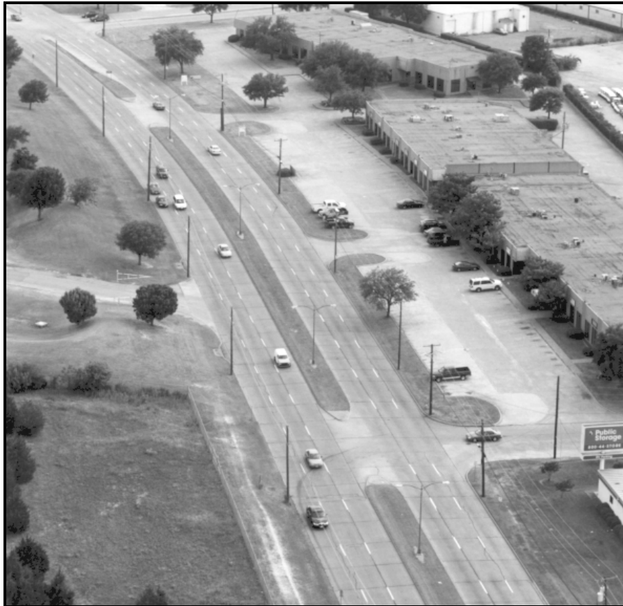
Figure 3-10. Unsignalized Access in Dallas, Texas.
