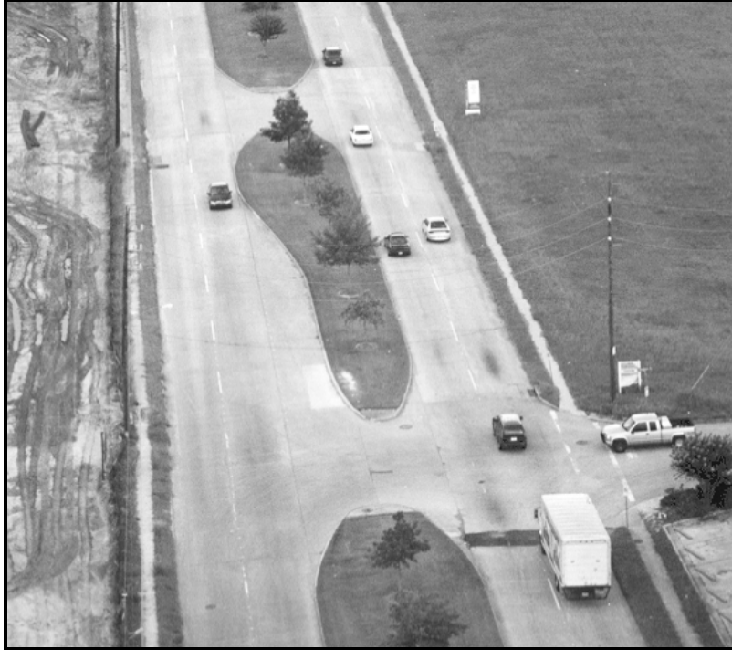
Figure 3-17. Full Median Opening (undeveloped area) in Houston, Texas.
