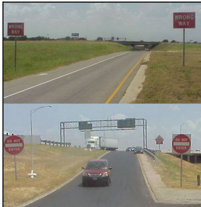
Figure 6. TxDOT Typical Gatepost Signing with the DO NOT ENTER and WRONG WAY Signs Mounted at Standard MUTCD Mounting Height.
