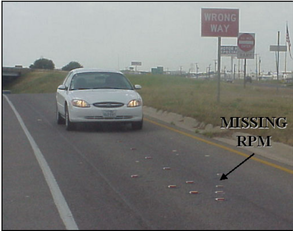
Figure 4. Wrong-Way Arrow with Missing Raised Pavement Marker.
